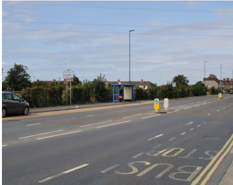
01: Old Shoreham Road
