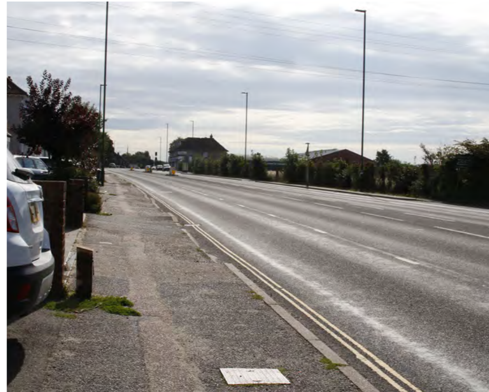
02: Old Shoreham Road
