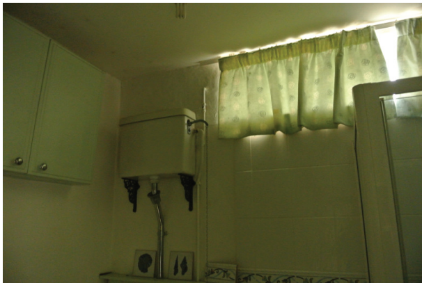
Fig 2.7 Bathroom with high level window
