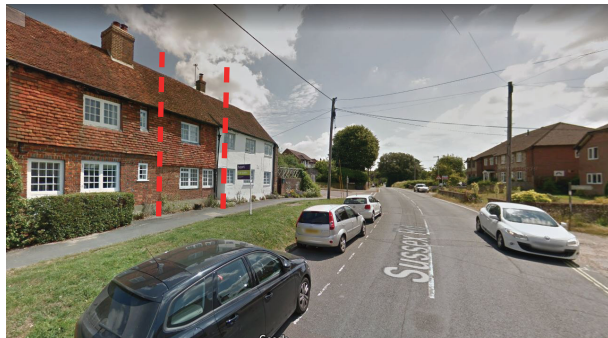
Fig 2.1 View from the West looking East along Sussex Road; no.24 on the left
