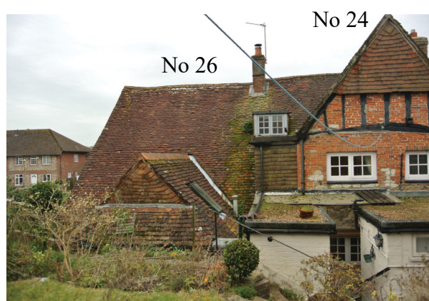
Fig 2.4 Rear of no.24 Sussex Road with no.26 Roof and no.26 dormer on the left
