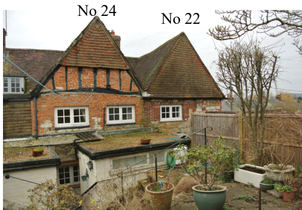
Fig 2.3 Rear gable and 1970's extension of no.24 Sussex Road; no.22 gable on the right
