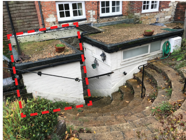
Fig 2.6 1970's rear extensions (extension on left outlined in red to be removed)
