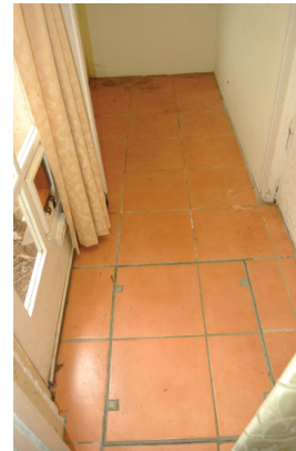
Fig 2.9 Existing narrow pantry
