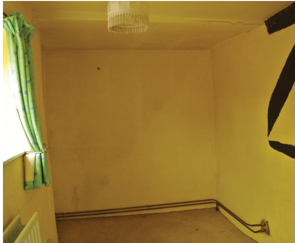
Fig 2.17 Bedroom 2 pipework to be rerouted beneath modern floor
