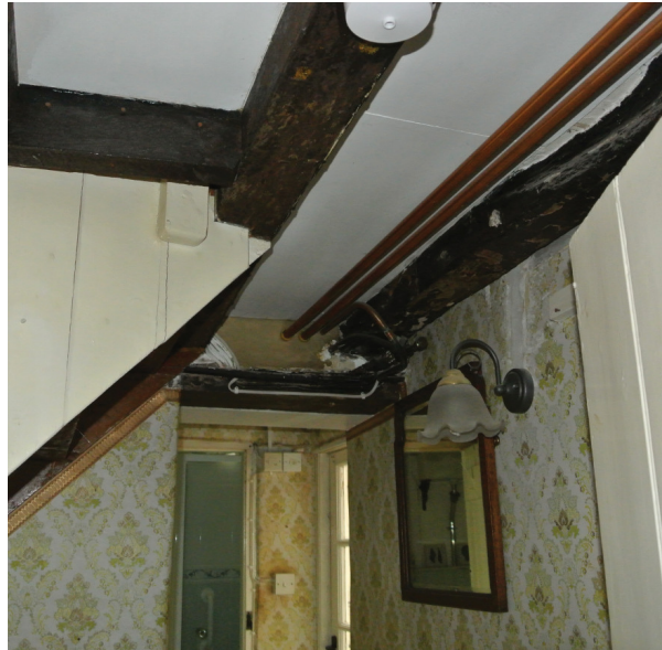
Fig 2.11: Pipework & cabling in existing hall. 1970's staircase on left
