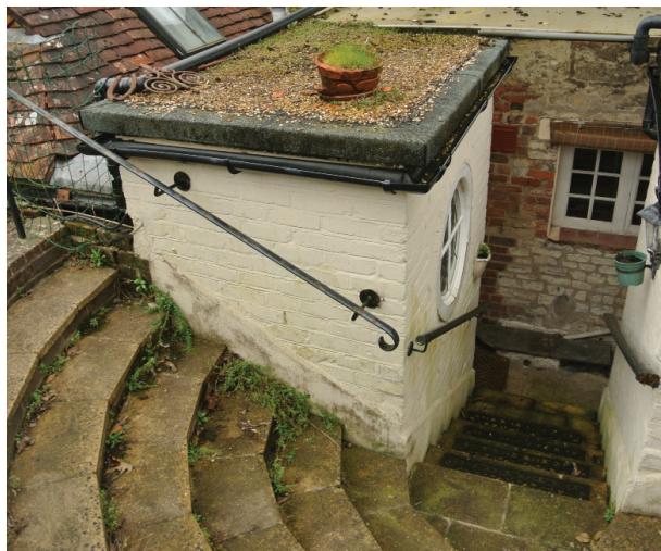
Fig 2.5 1971 pantry extension to be removed; stone and brick infill visible behind on the rear elevation of the older part of the house
