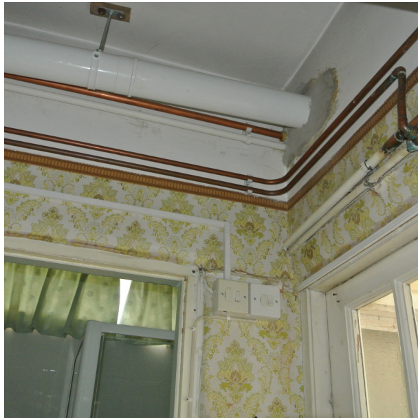
Fig 2.4 Ceiling in rear lobby showing pipework and conduits
