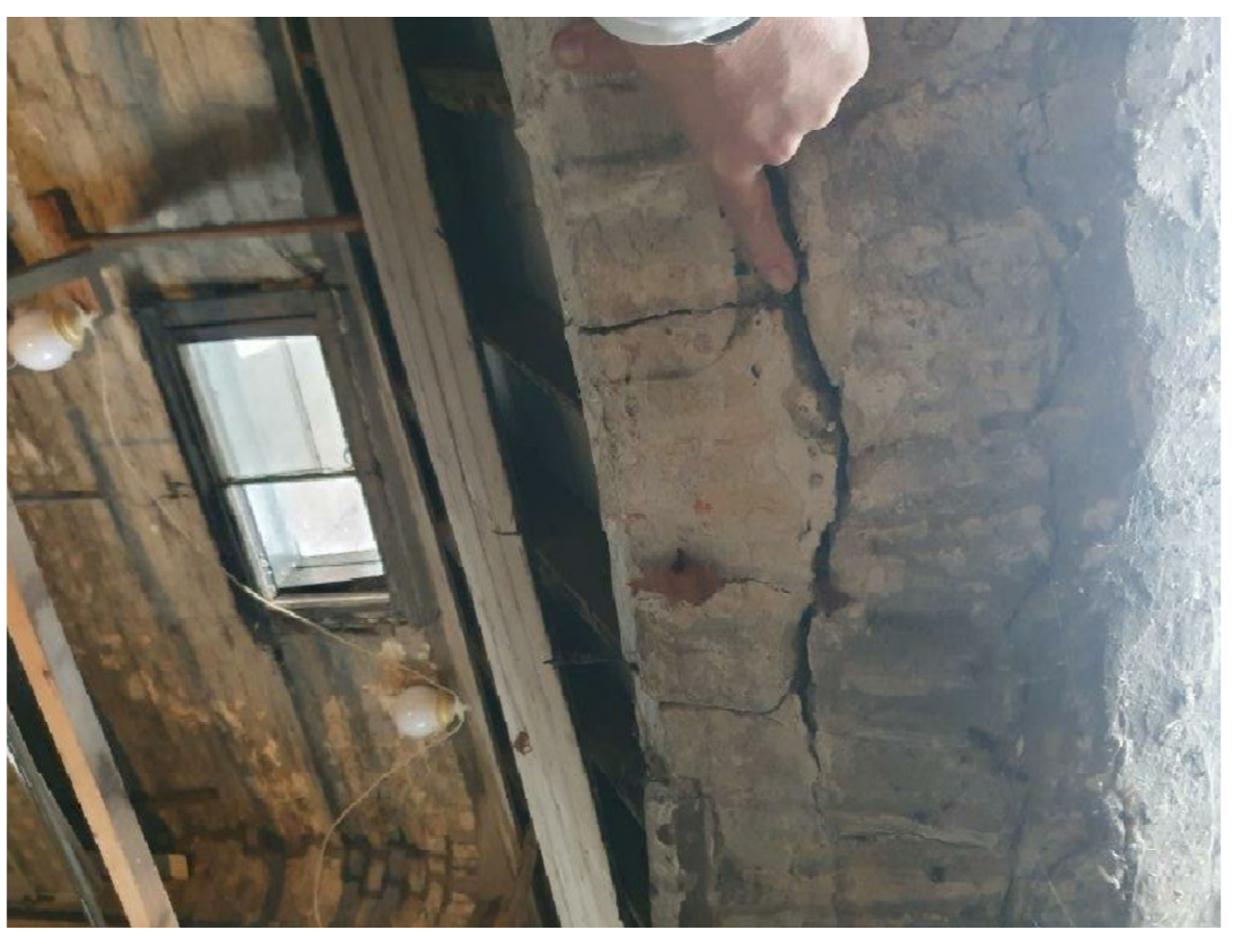
Structural crack internally - Rear wall
