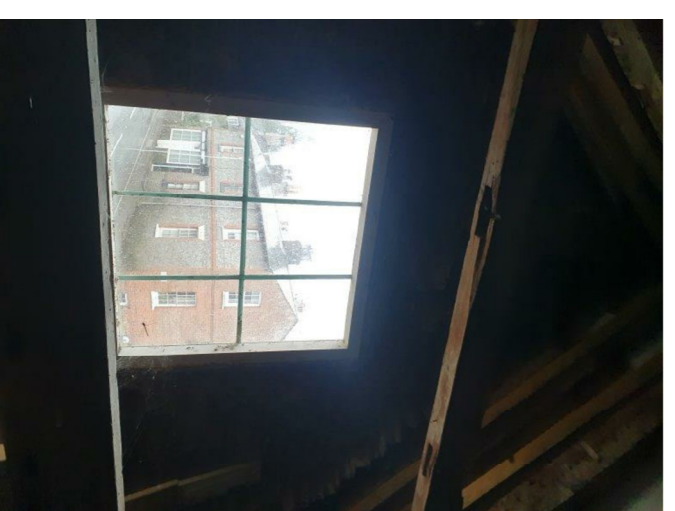
Gable above arch - poorly supported
