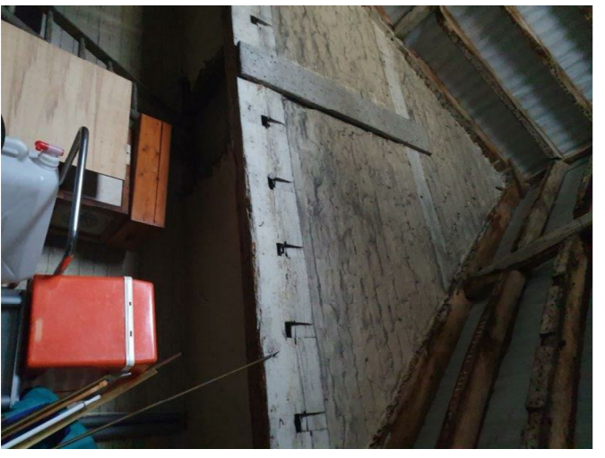
Check gable to bedroom five
