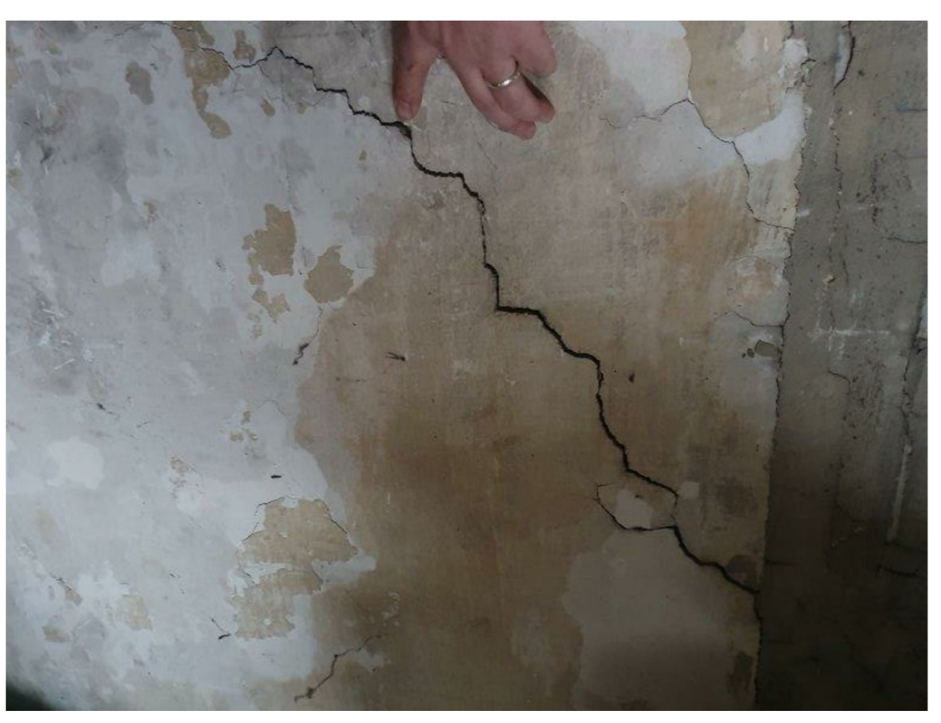
Close up of structural crack internally - Rear wall indicating downward/sideways movement of above structure
