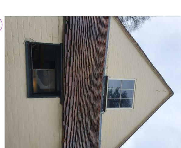
South gable elevation with sagging mono pitch roof, bulging of wall below roof and structural cracking to bottom left of window.
