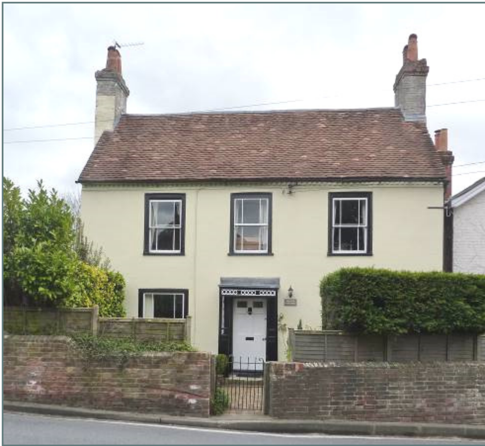
Figure 22: Millers Cottage , High Street: Early 19 th century. Grade II listed for group value.
