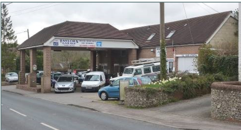
Figure 14: Taylor's Garage represents a visual intrusion into the street scene. Should, in time, the current use ever cease, its sympathetic redevelopment with a high quality design could represent a significant opportunity to enhance the Conservation Area.
