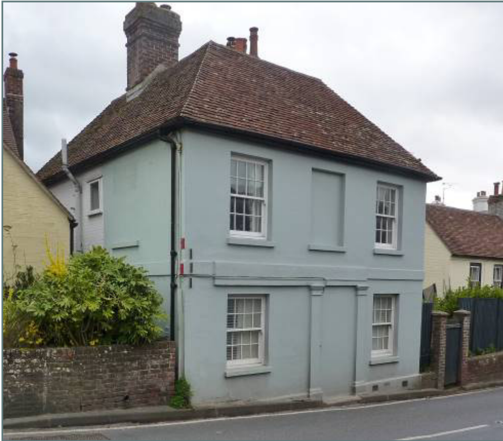
Figure 20: The Old Post House. The pilasters, blocked door and mutilated cornice are the remnants of an earlier shopfront.
