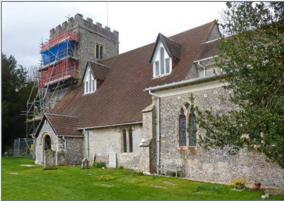
Figure 33: The south elevation of the church has unusual 19 th century dormers and evidence of a 'classicizing' phase in the building's history. The building features on Historic England's Heritage at Risk Register and is subject to a repair programme.
