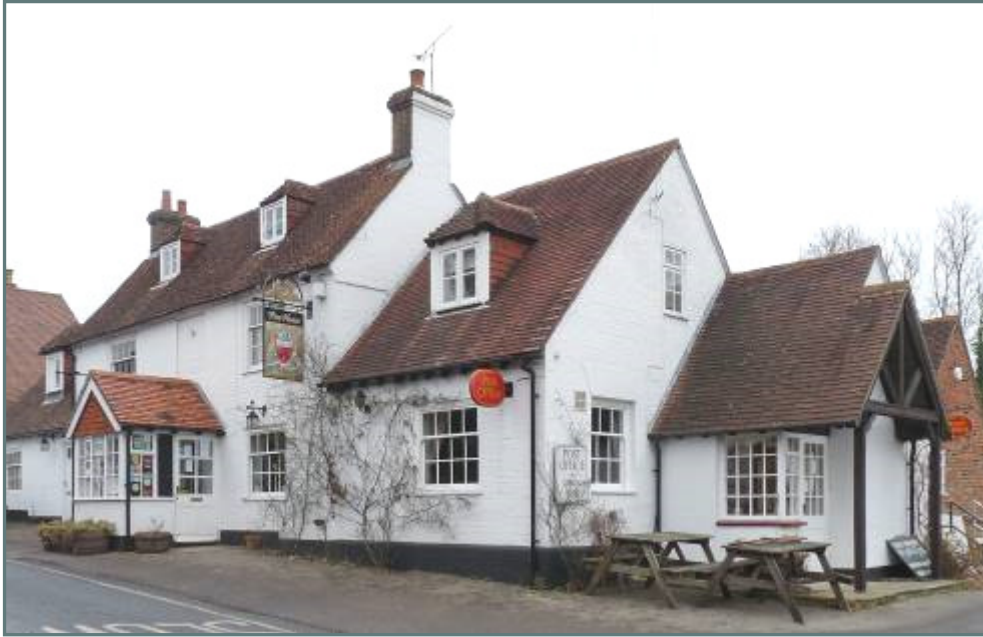
Figure 15: The Bakers Arms , High Street: originally an 18 th century house, later converted into a public house. Grade II listed. Also accommodates the Post Office. Some tidying of the area around the pub would enhance its setting and the wider Conservation Area.
