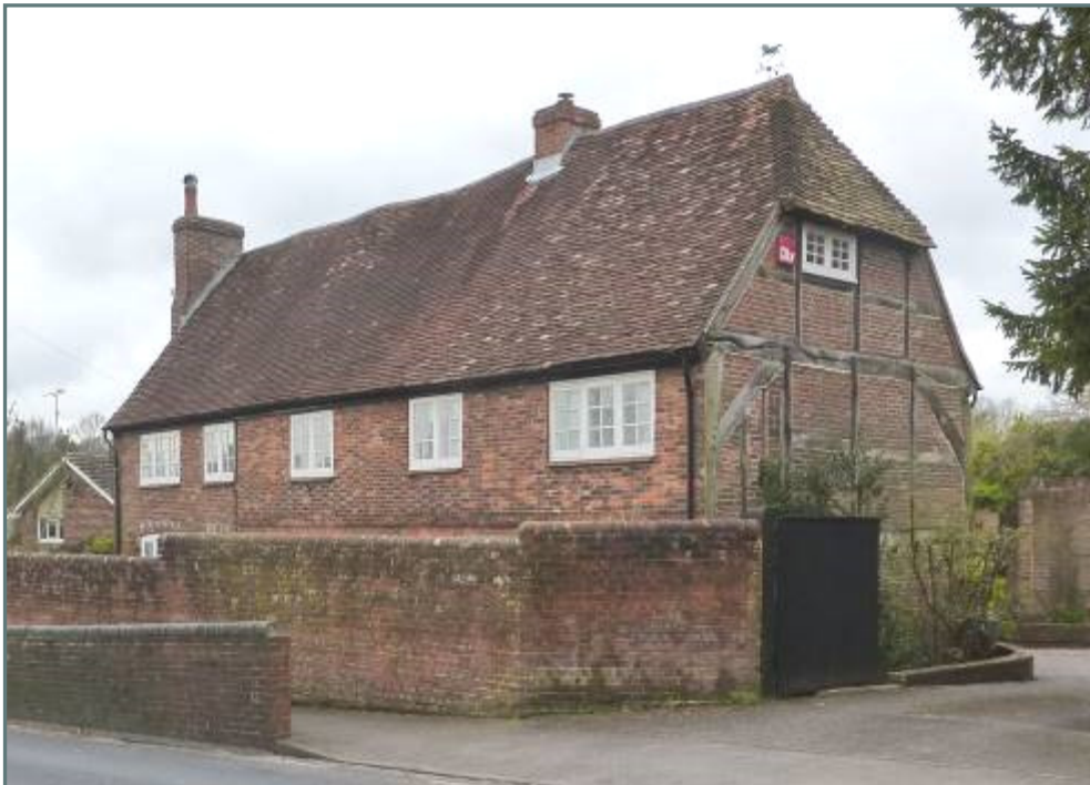
Figure 16: The Small House , High Street: a 16 th century timber frame with 18 th century re-cladding and early 19 th century extension. Grade II listed.
