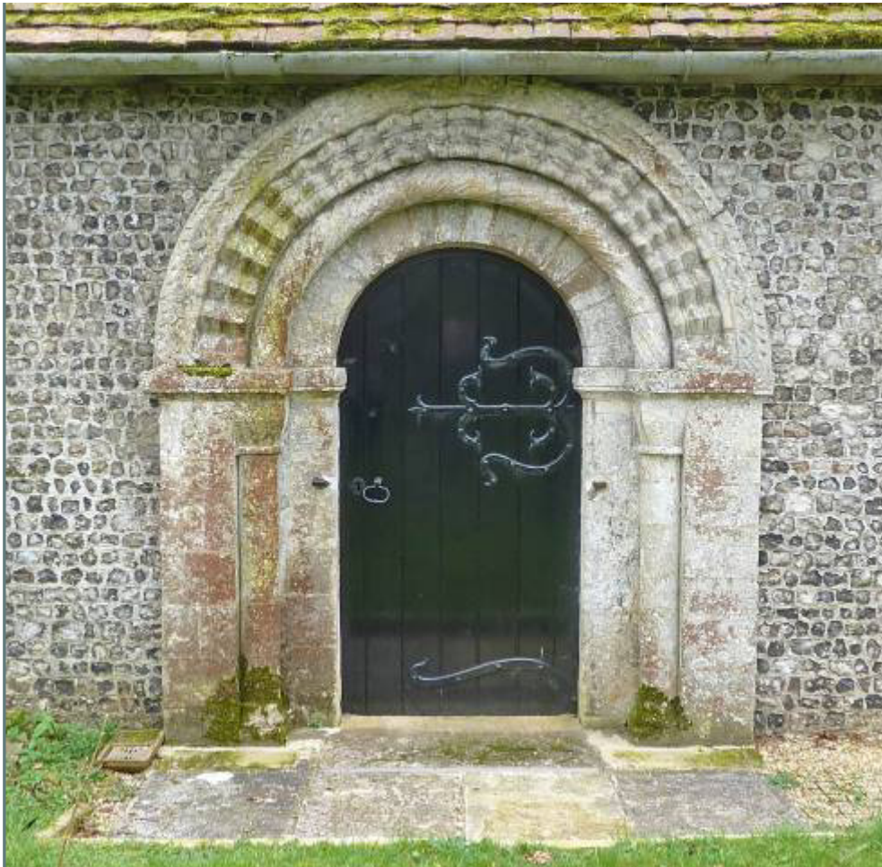
Figure 34: Romanesque door on the north elevation of the church
