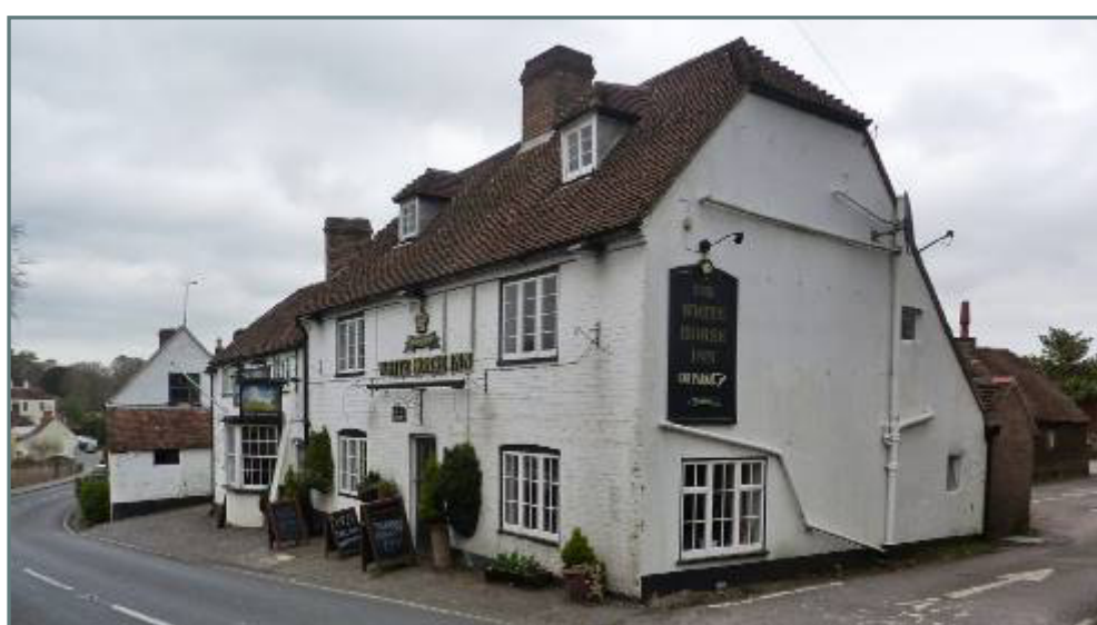
Figure 44: Willow House , South Hill. Late 17 th century with early 19 th century features and additions. Grade II listed.
