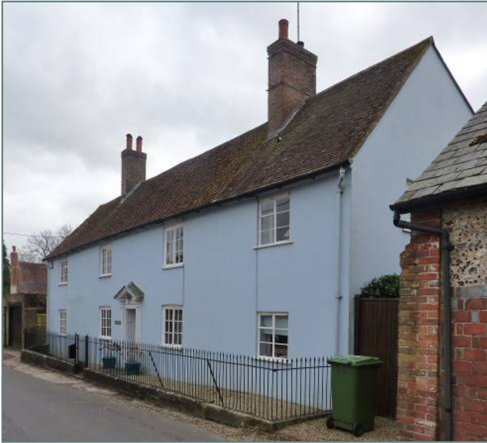
Figure 41: Clarks House , Park Lane. Recommended as a 'Locally Listed building' in the Management Plan
