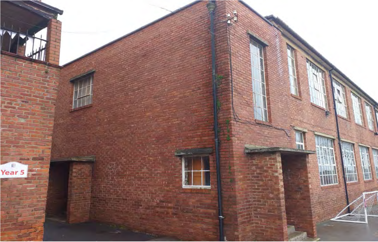
Photograph 2 – Southwest corner of existing dining hall.
