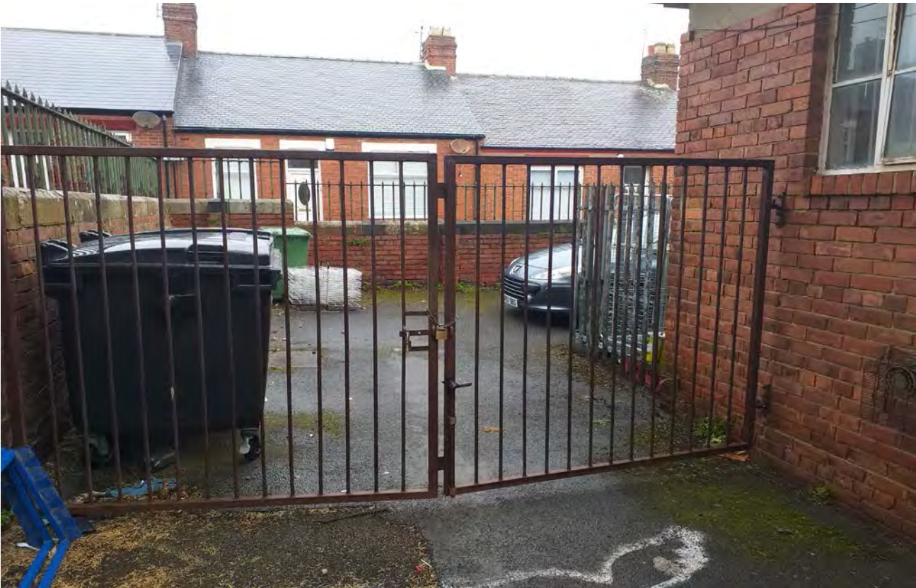
Photograph 1 – Access to the hall from the northern site area.
