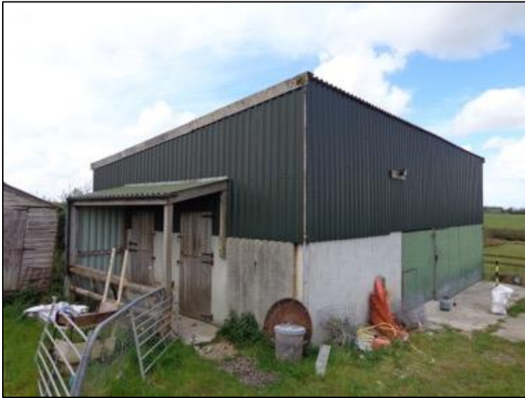
Figure 1. Barn viewed from the south-east
