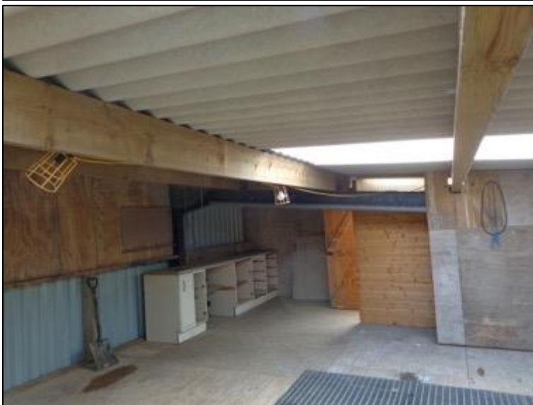
Figure 2. Interior view of barn
