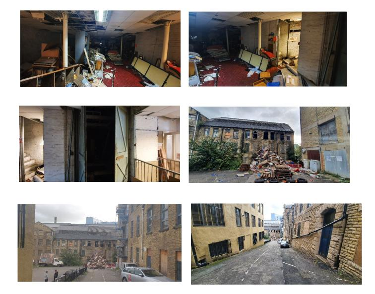
As per above images, the condition of the existing building will need full repair, and renovation, from re-pointing, to new timber windows, new roof, new flooring, new stairs.
