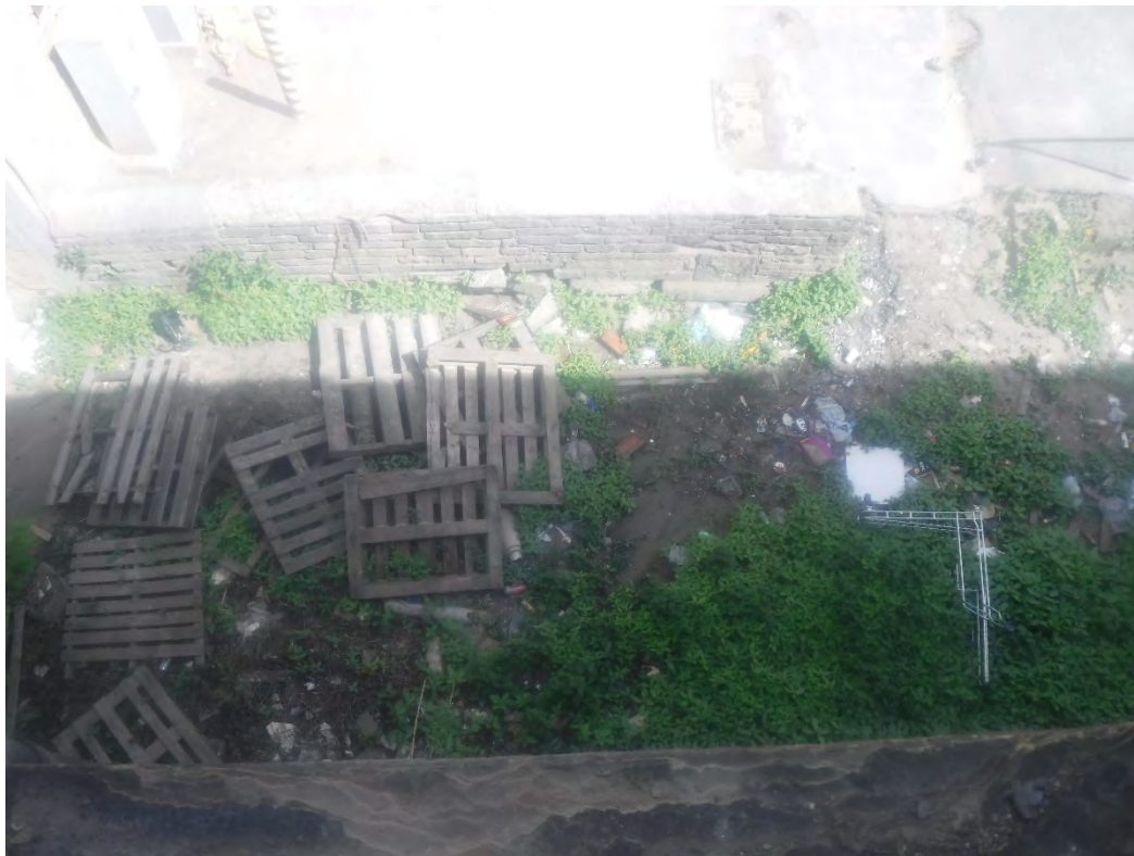
Photograph No.9: View from second floor window of northern boundary
