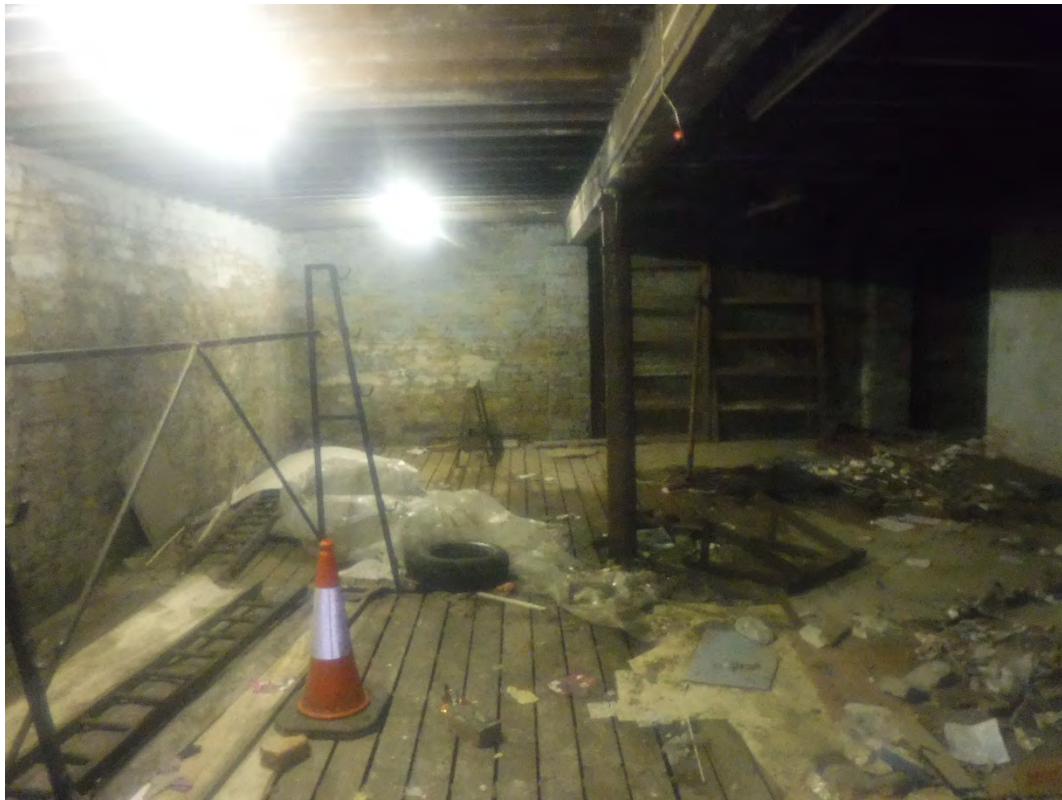
Photograph No.4: Basement level
