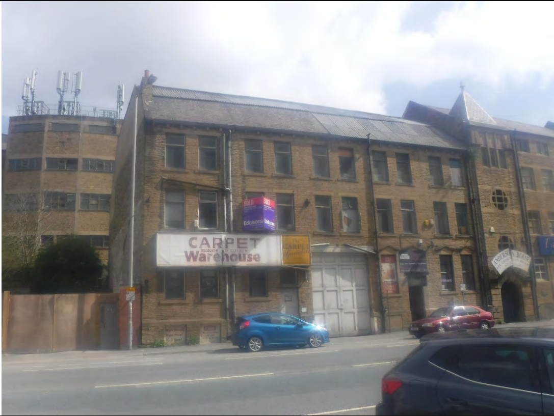
Photograph No.1: View of site building from Thornton Road looking north
