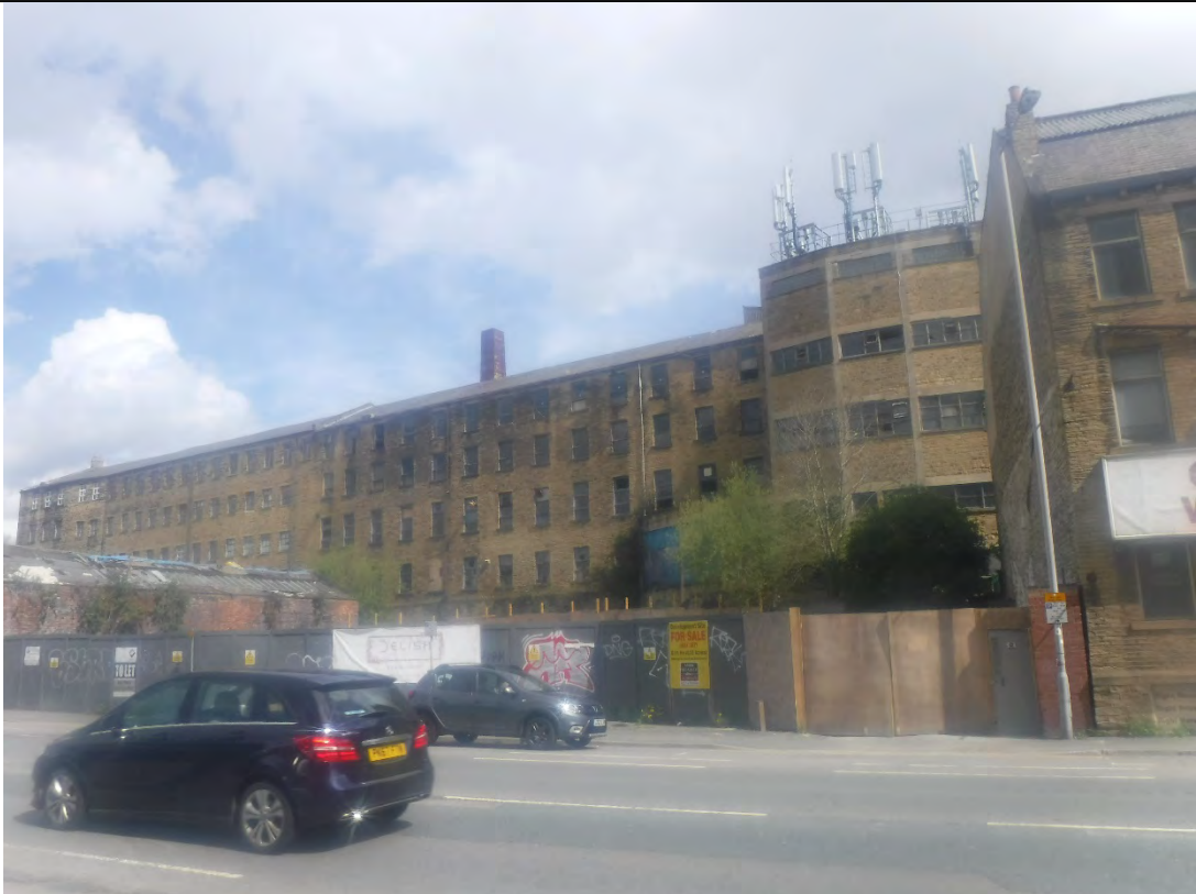
Photograph No.2: Cleared ground to west of site behind roadside fencing
