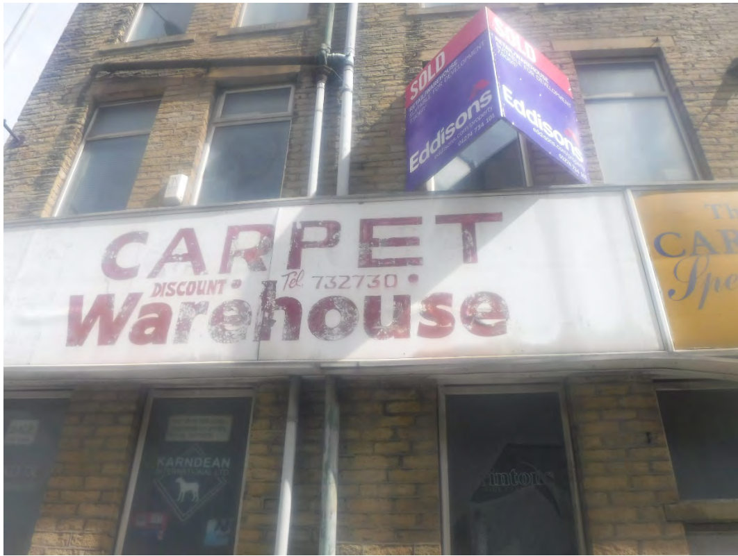
Photograph No.3: Closer view of front of site structure
