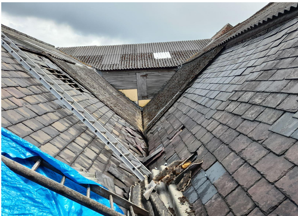
Plate 4: Another photograph showing lifted and missing roof tiles.
