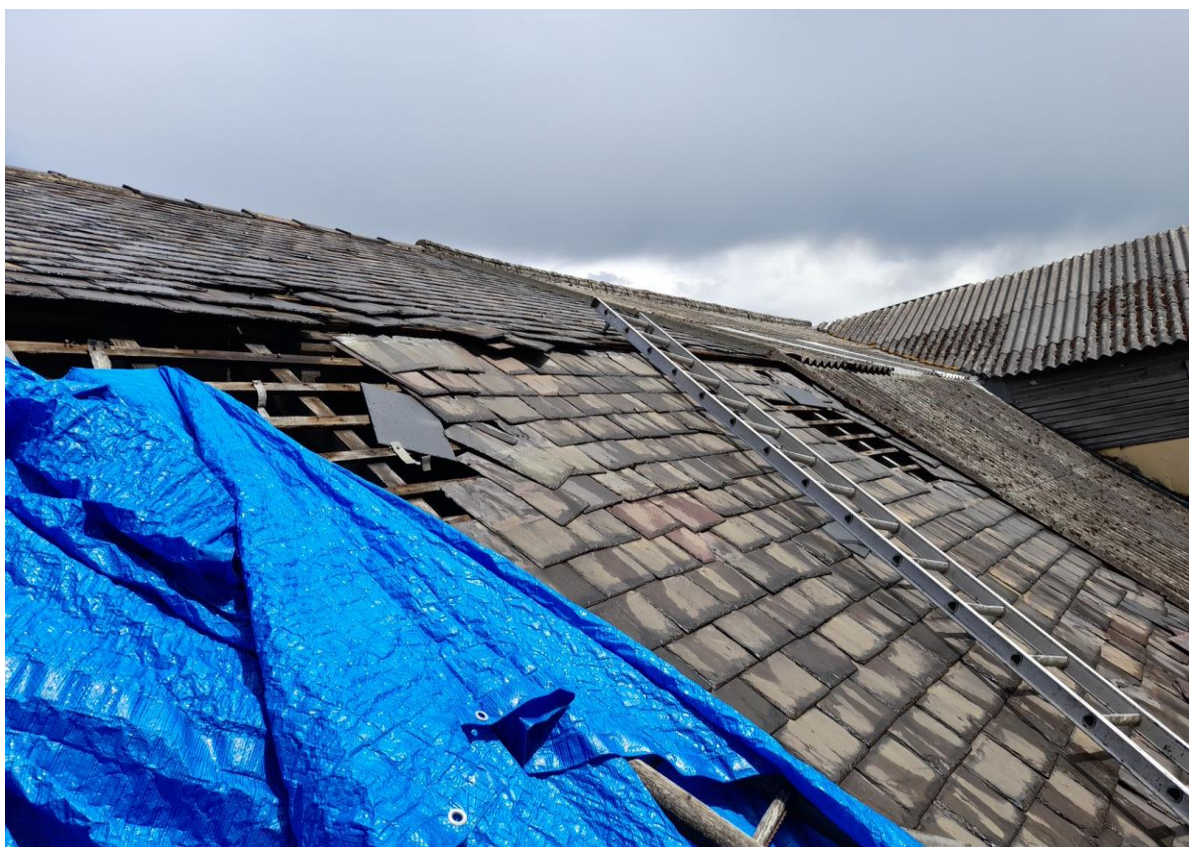
Plate 4: Another photograph showing lifted and missing roof tiles.
