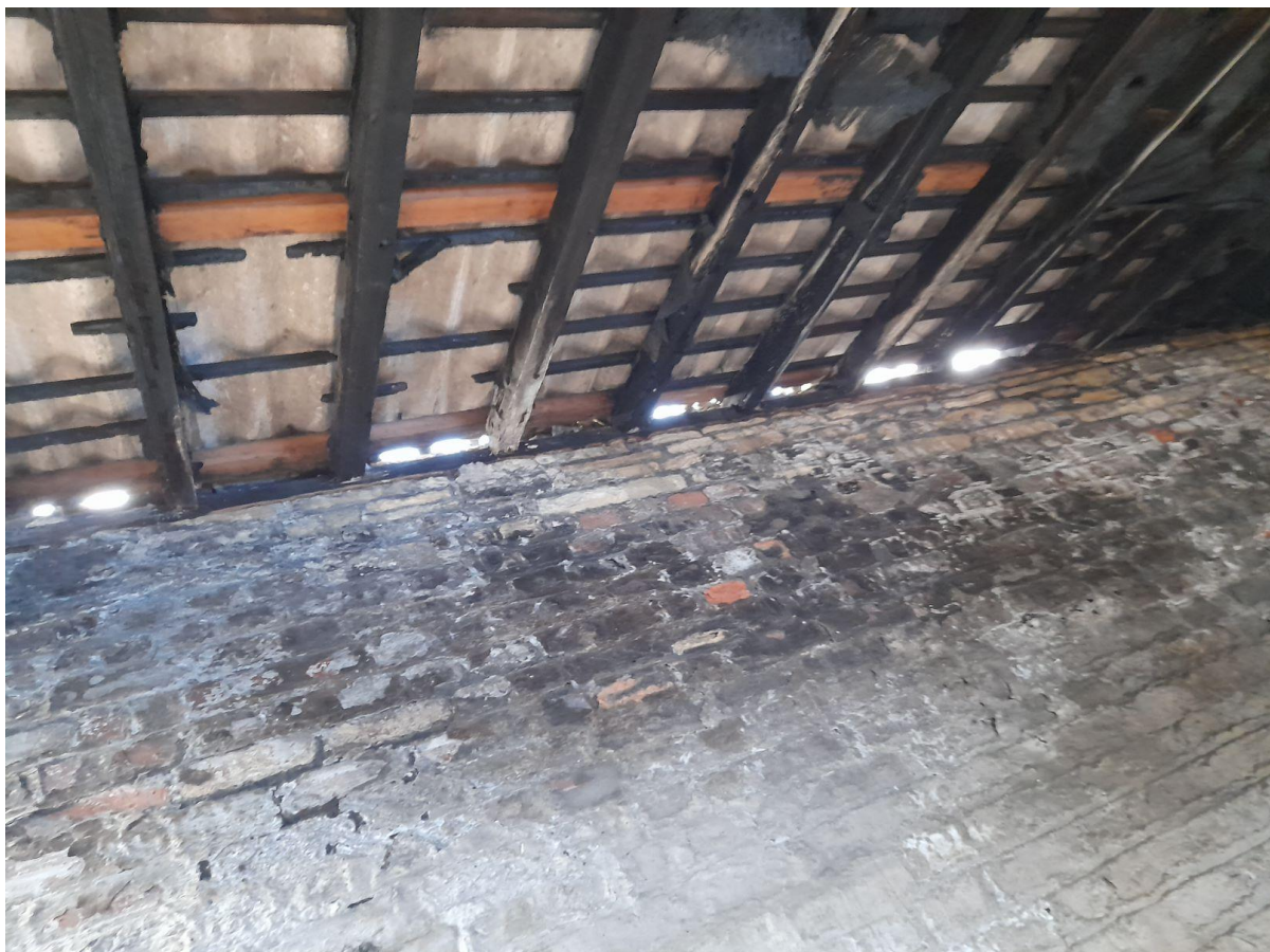
Plate 7: An image showing the gaps between the roof and walls.
