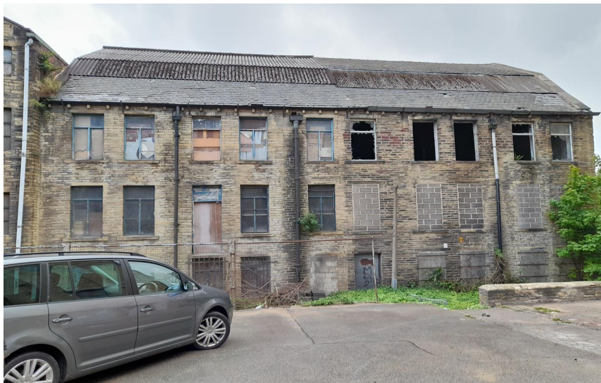
Plate 2: An image showing some of the missing/ lifted tiles and broken windows.
