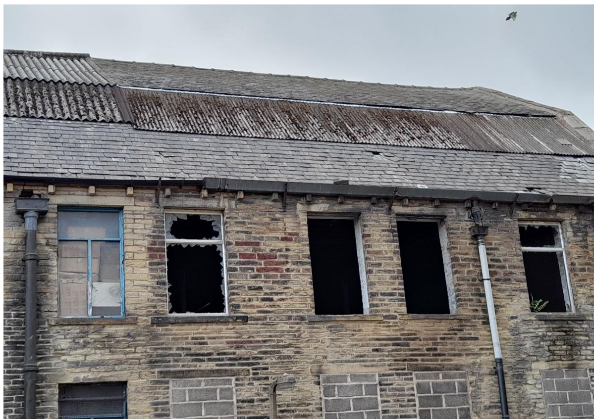
Plate 2: An image showing some of the missing/ lifted tiles and broken windows.
