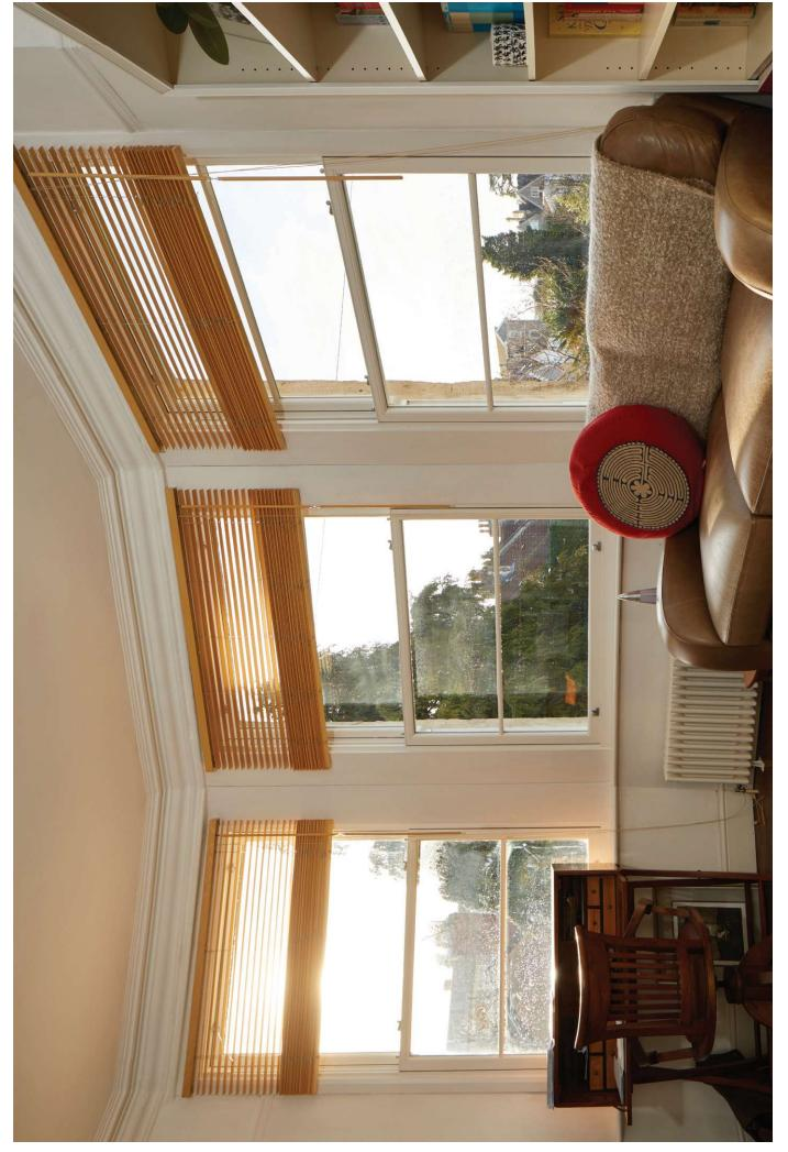
The system has two sashes built into the frame which slide in opposing directions and will remain fixed in any position.
