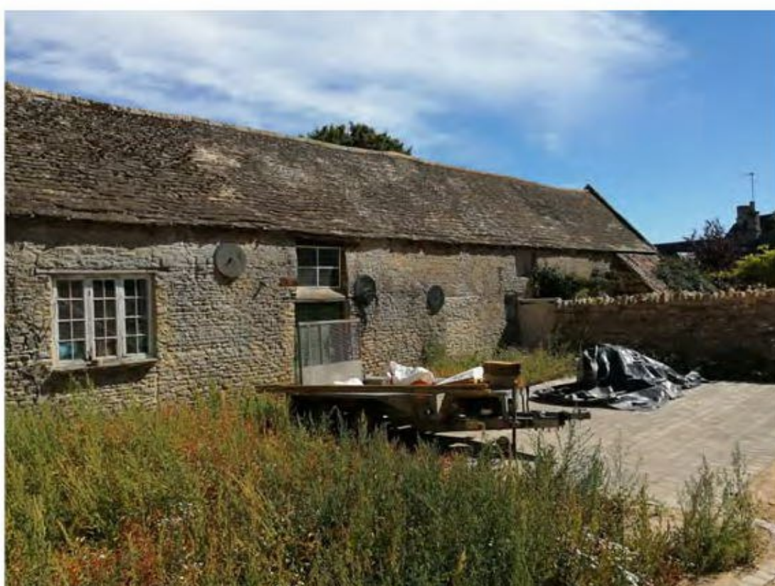
Plate 2 Looking South East Along Barn
