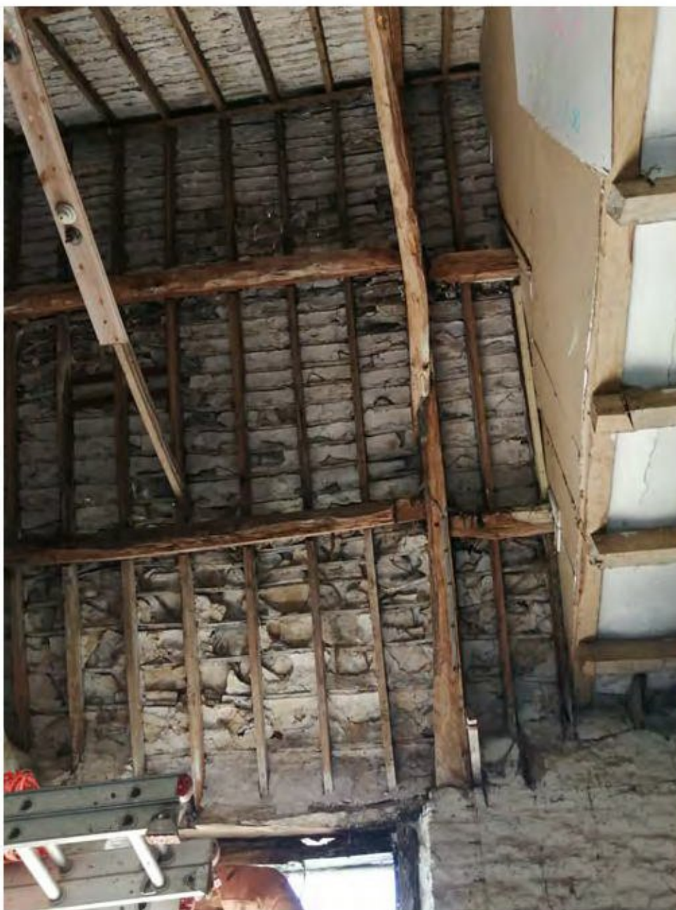
Plate 13 Looking at Roof Structure above Workshop
