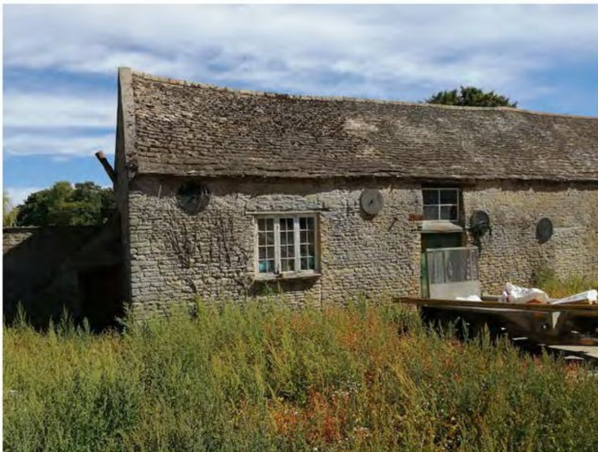
Plate 1 Looking East at West Elevation Indicating Undulating Roof Line & Tie Rods
