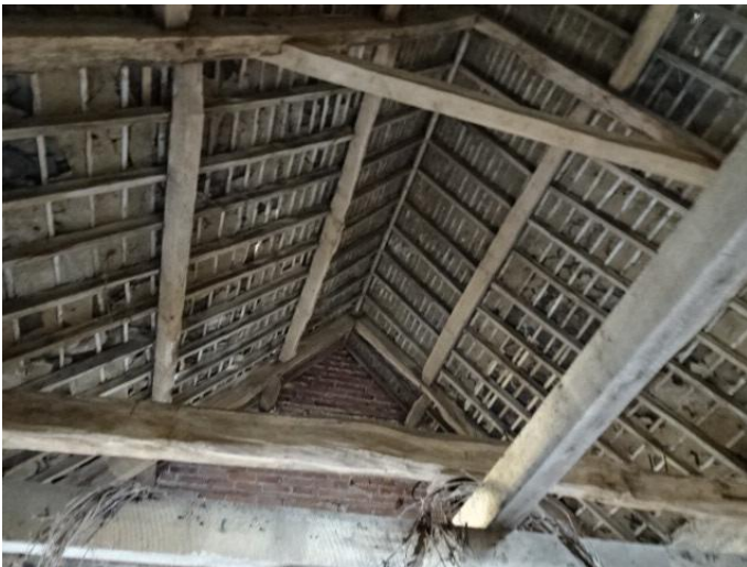
Barn roof structure (south section)
