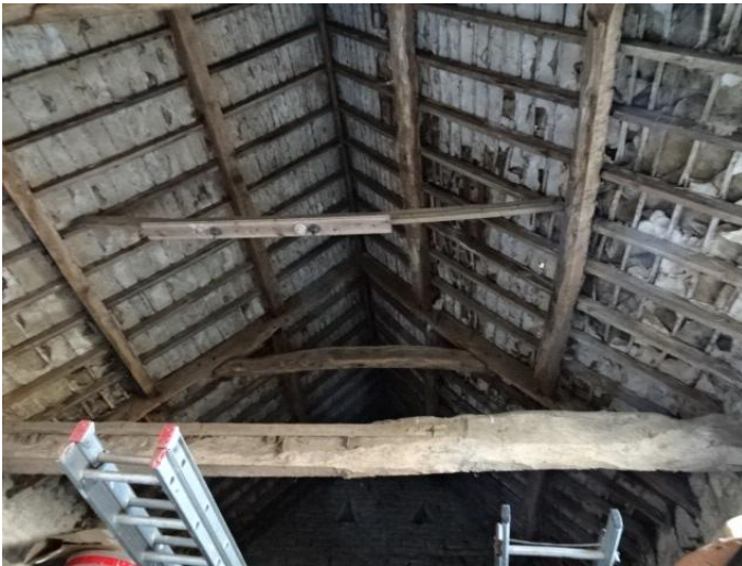
Barn roof structure (north section)
