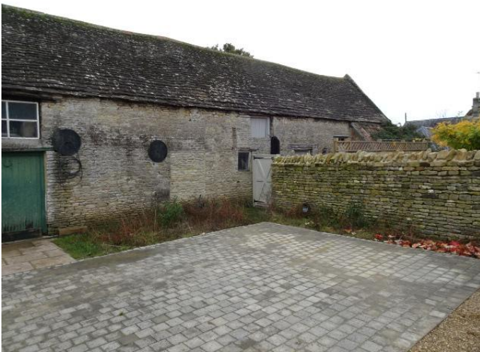
Part of west elevation from Estate Yard
