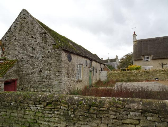
General view from northwest of barn
