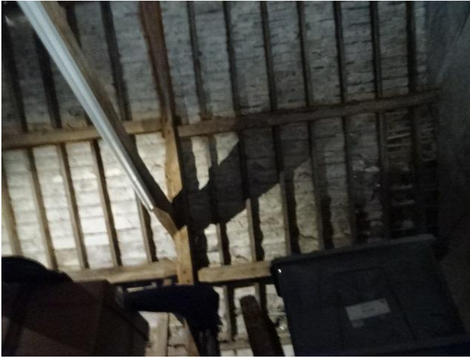
Barn roof structure (middle section)
