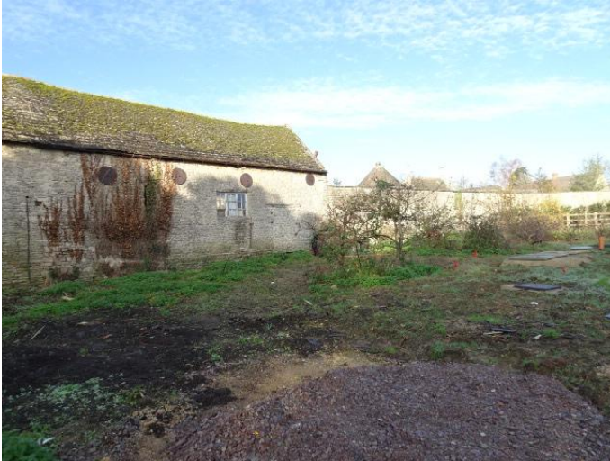
East elevation from kitchen garden
