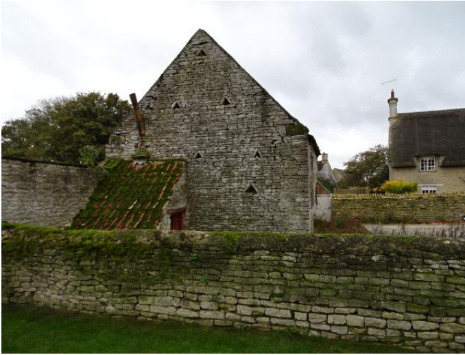
North gable end
