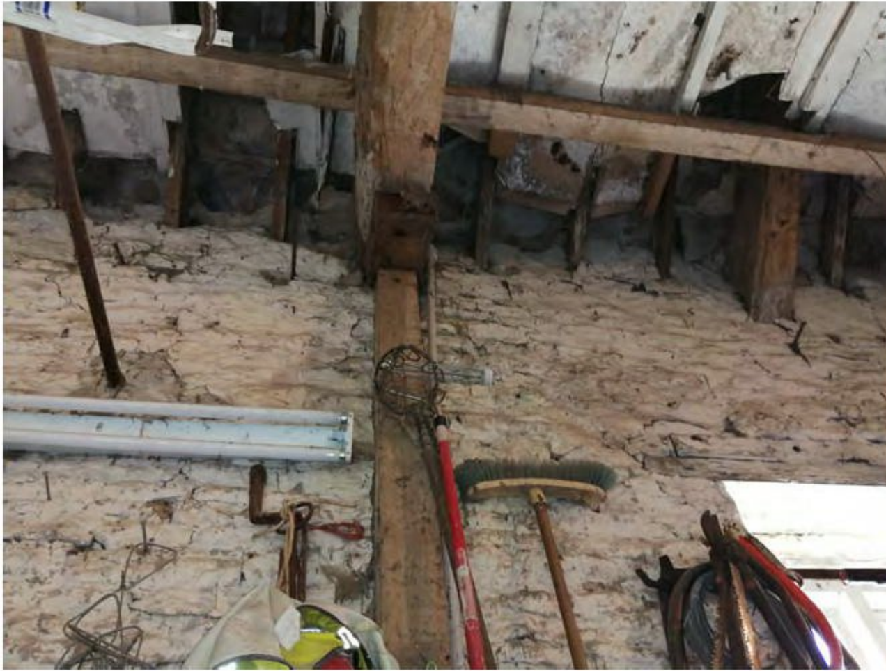
Plate 14 Looking at Reduced Bearing to Truss to Workshop
