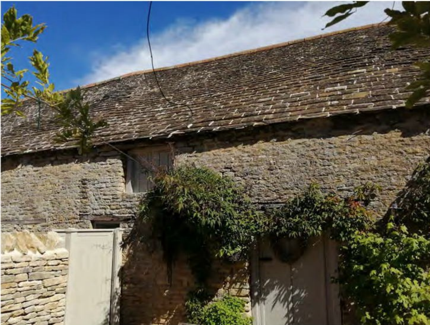
Plate 5 Looking East at Roof Structure With no Rainwater Goods Present
