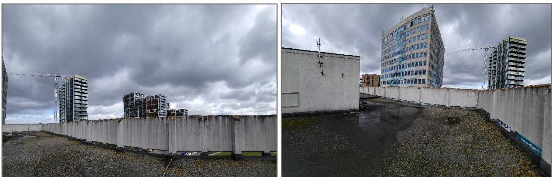
Images from the 4 th floor roof of Riverside House. Neighbouring buildings visible but no direct view of any rooftop plant or any audible plant.
