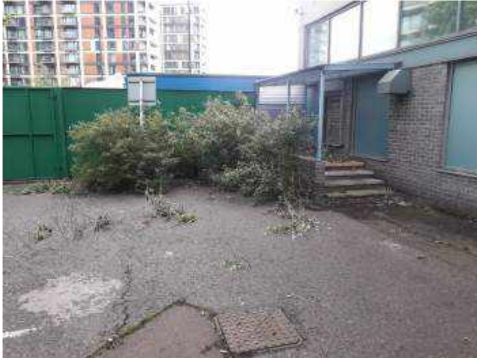
PHOTO 1: External area of the site within hoarding showing overgrown vegetation.
