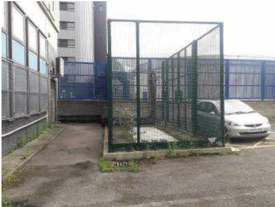
PHOTO 6: Location of the former fuel generator within the side car park.
