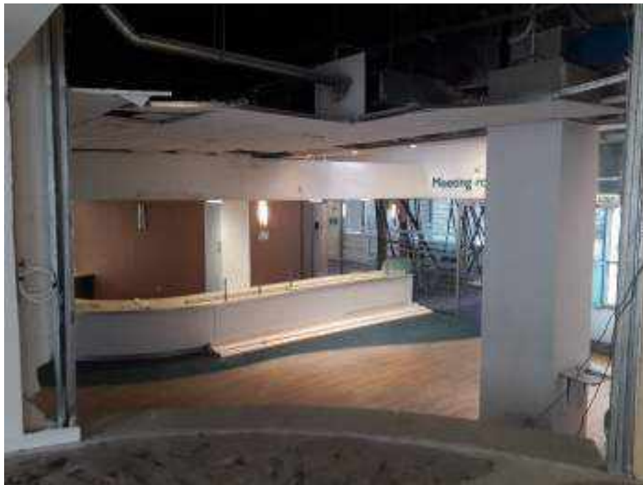
PHOTO 4: Overview of the ground floor main foyer.
