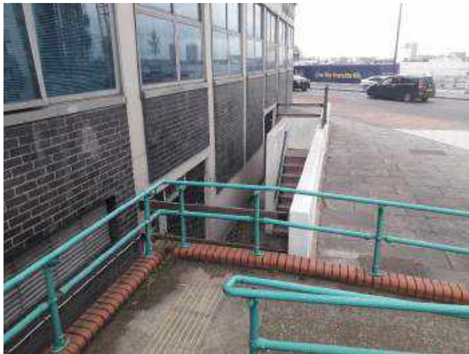
PHOTO 2: Overview of the undercroft area to the north of the site where the electricity substations, boiler room and telephone room are accessed from.
