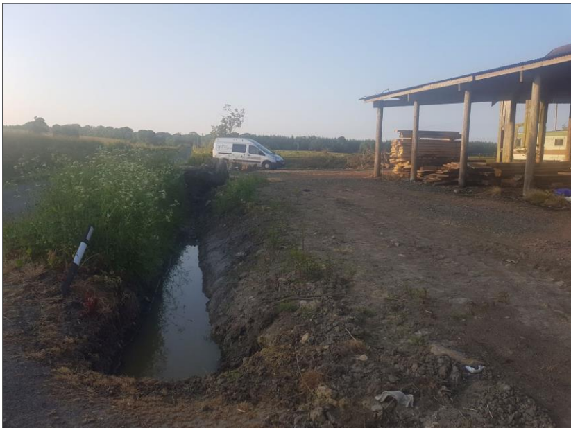
Figure 8. Man-made ditch to west of the building.
