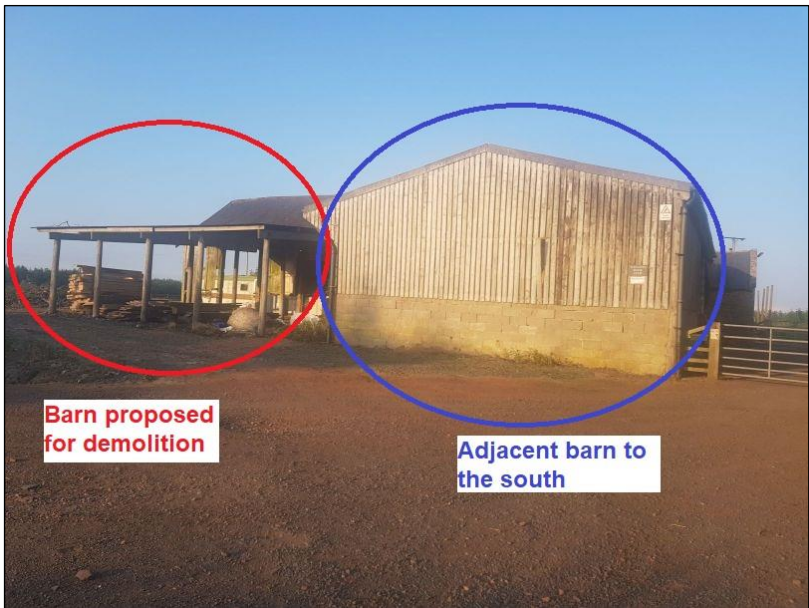
Figure 12. Annotated image showing proximity of adjacent barn to the south.
