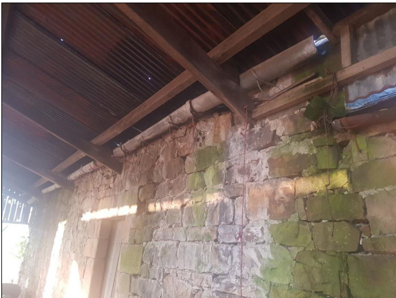
Figure 9. Eastern elevation abutting stone building.
