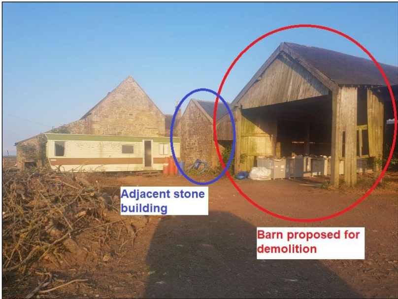
Figure 13. Annotated image showing proximity of barn to the east.
