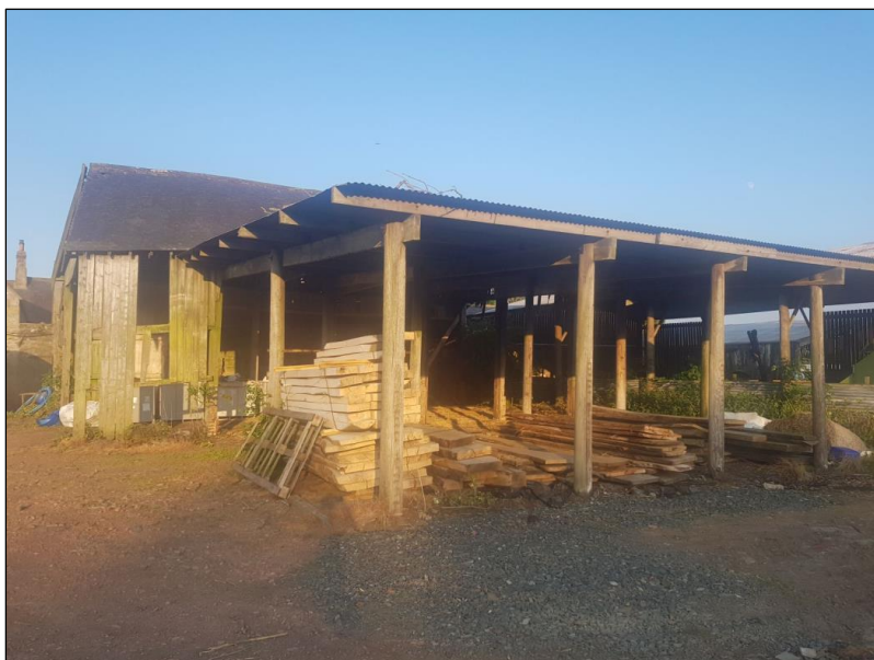
Figure 5. Building – northern and western elevations.
