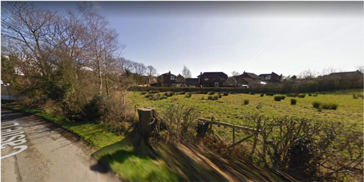
Figure 12: Picture of the eastern extent of the site prone to flooding (Source: Google Maps, 2021)
