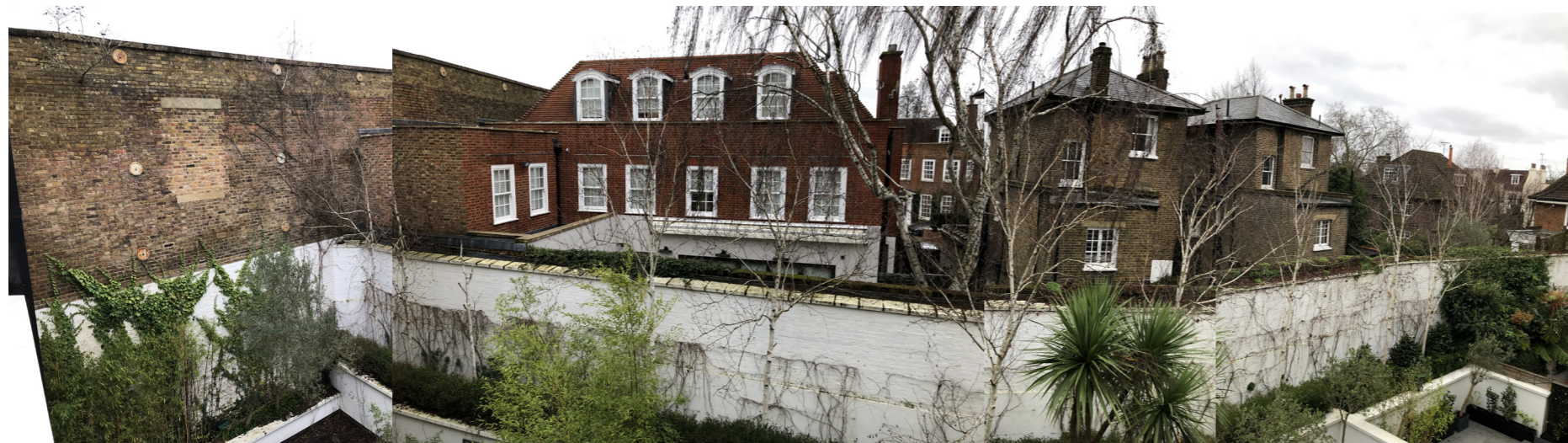
View from first floor rear, with high boundary wall to St John's Barracks on the left, no. 7 and no. 9 Acacia Place the otherside of the rear boundary wall.
