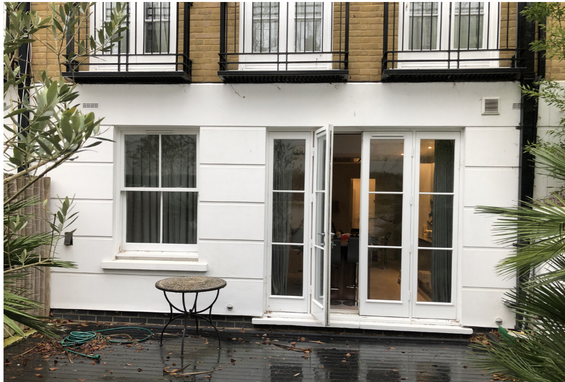
Existing rear elevation of no.7
