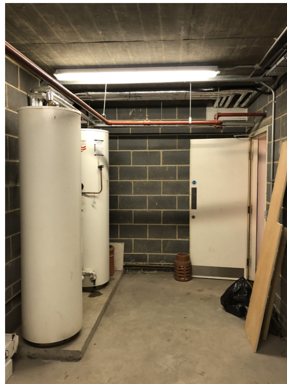
Existing basement plant / store room
