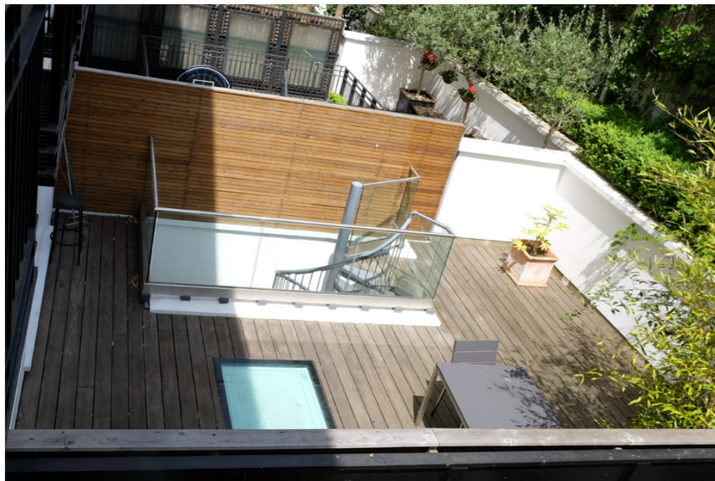
no.9 basement infill
