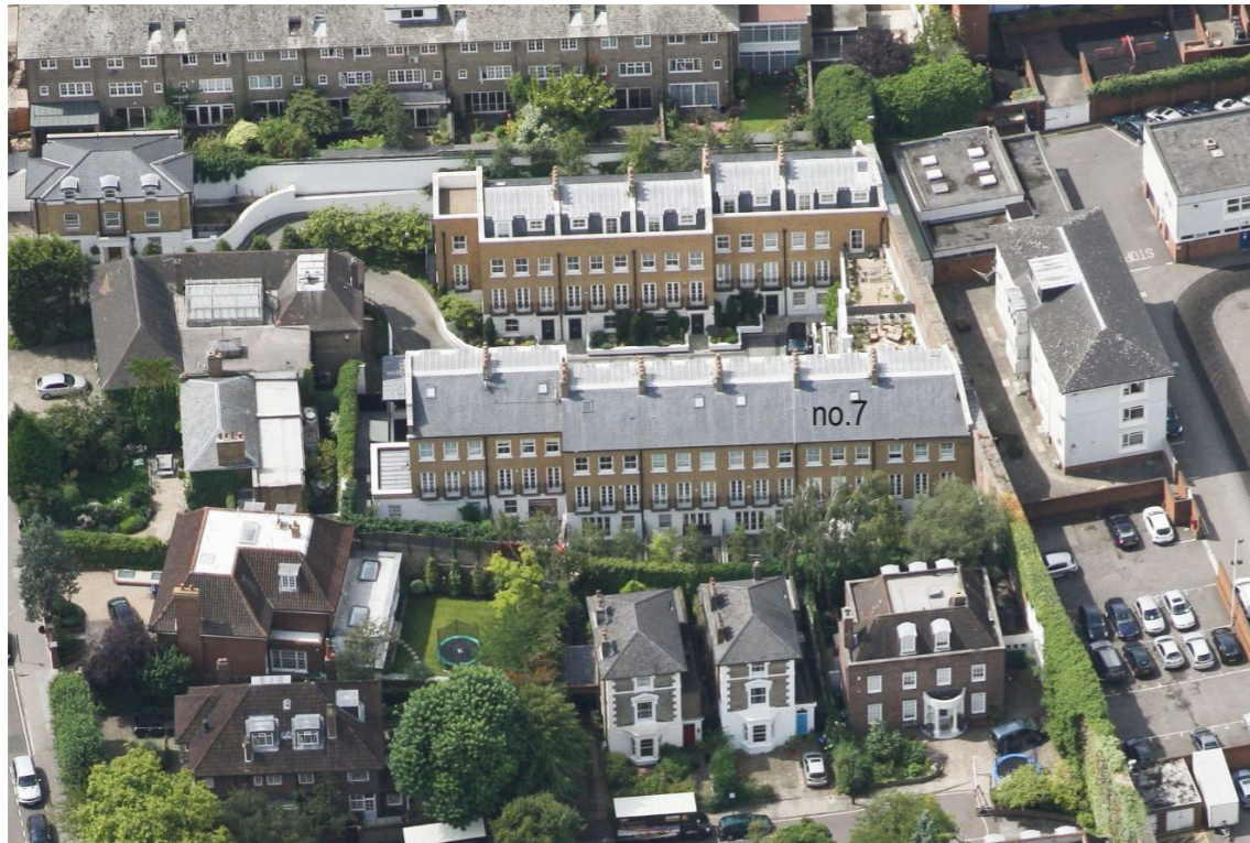
Aerial view looking west
