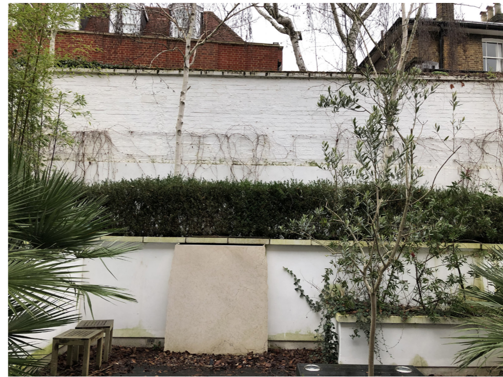
Existing tall rear garden boundary wall and planter
