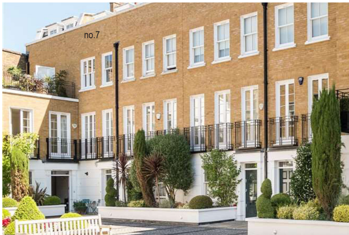
Existing courtyard, view looking northeast, with no.7 located in the left hand corner
