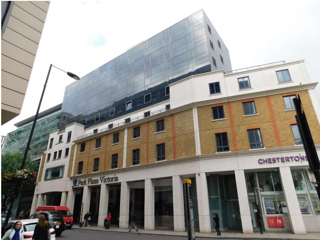
Figure 2. Photograph of host building (A)
