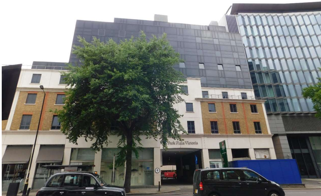
Figure 3. Photograph of host building (B)
