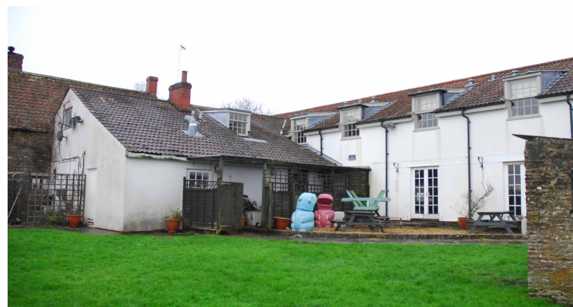
Figs. 4 The rear of the building in March 2020
