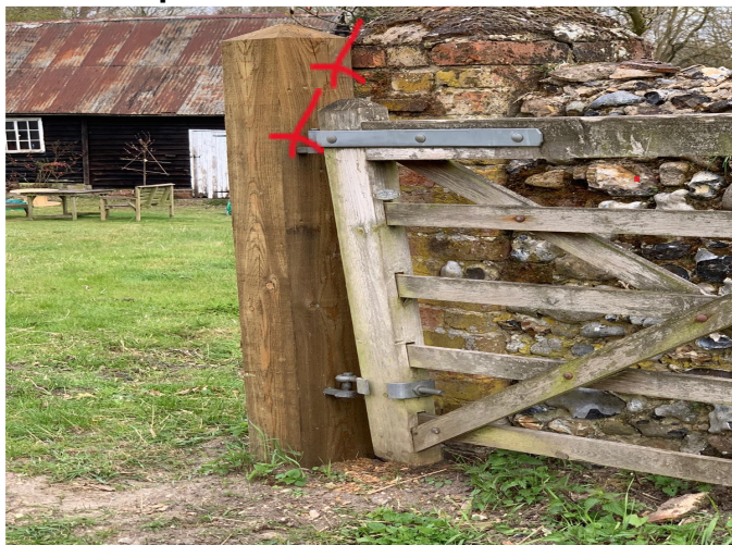
Photo 22 post weir socket to be fitted
