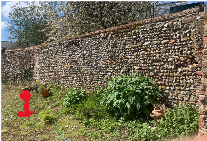
Photo11. Stone wall front
