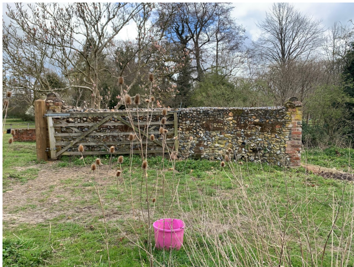
Picture 20 &21– side of stone wall surrounding magnolia tree
