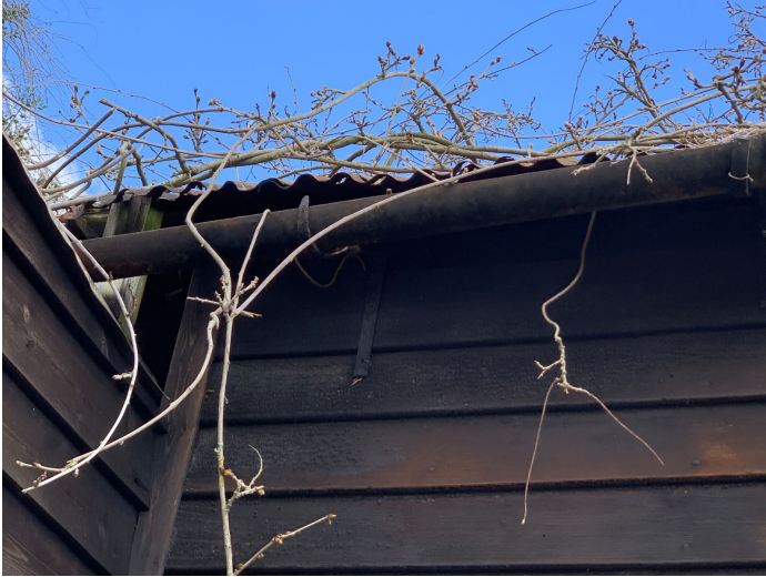
PICTURE 6: Roof and guttering and feather edge on outer house with needs repair.
