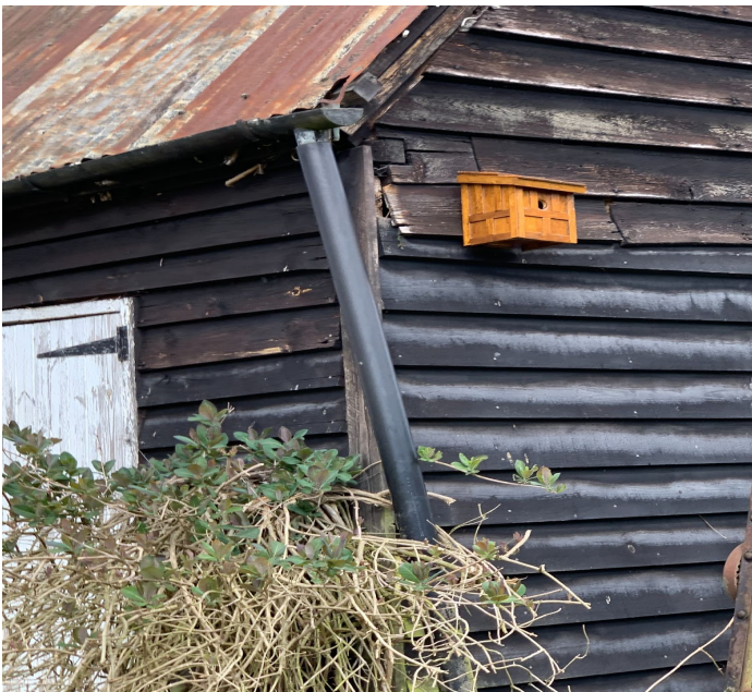
PICTURE 6: Roof and guttering and feather edge on outer house with needs repair.
