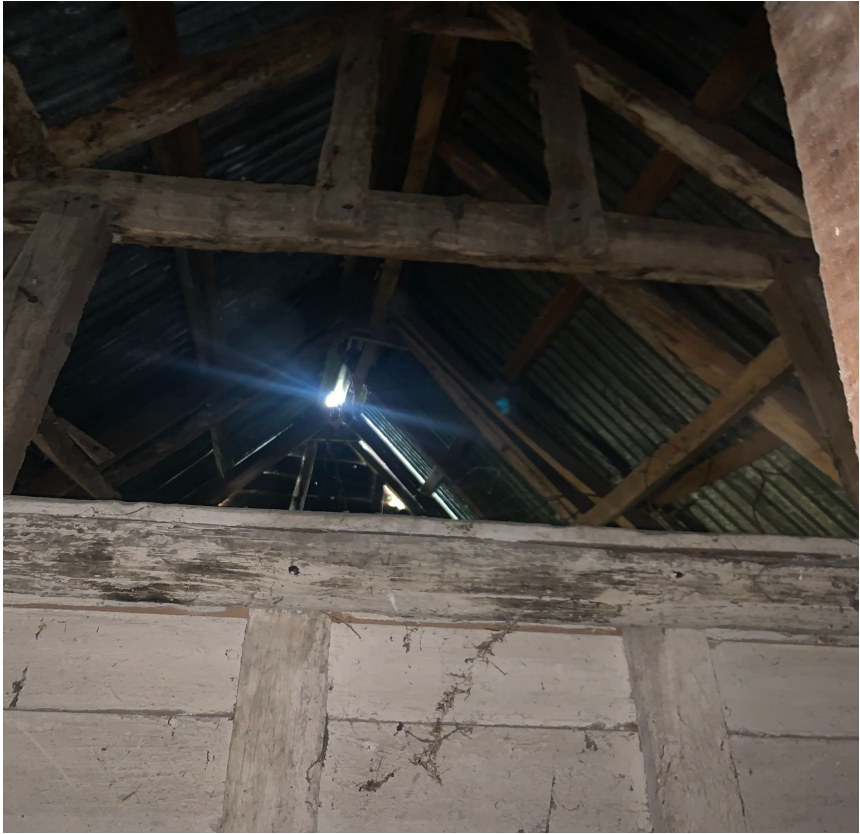
Photo 9: inside of outerhouse
