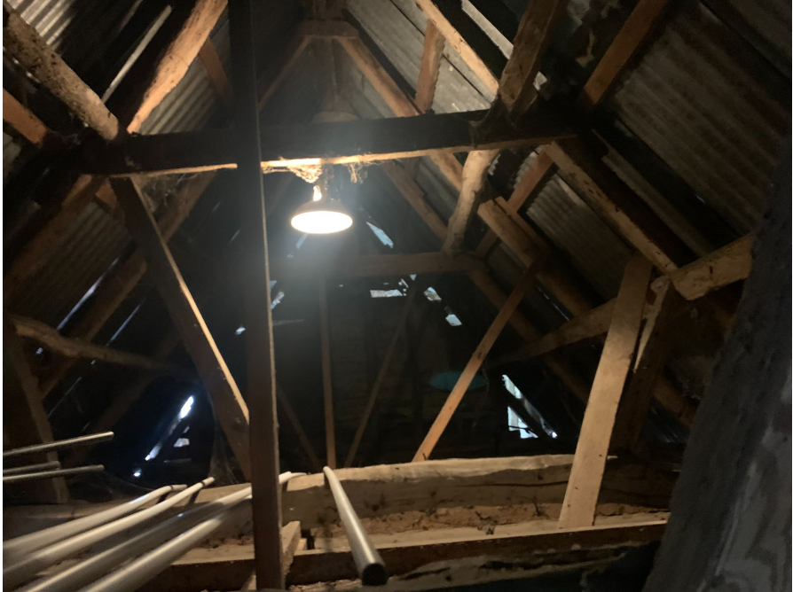
Photo 8: Roof inside of outerhouses
