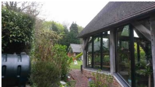
Figure 13 Rear view C20 extensions showing the existing oil tank Left
