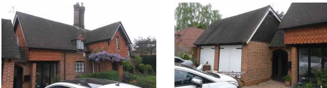
Figure 10 L West end of cottage and R. C20 garage
