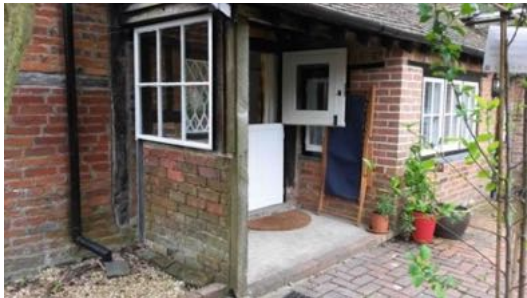
Figure 12 Rear view East End and C20 extensions
