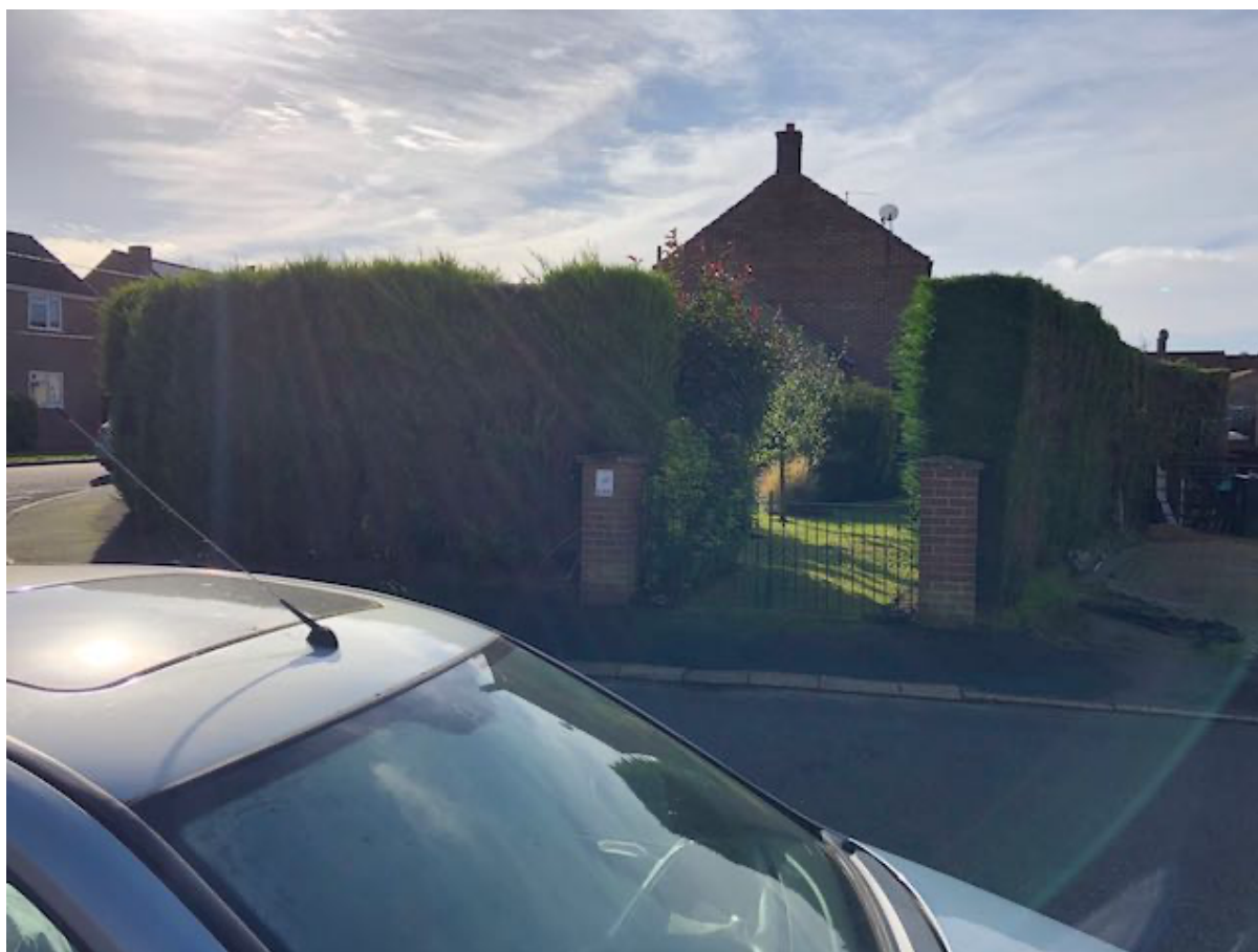
East elevation viewed from Forester's Avenue showing the existing vehicle access
