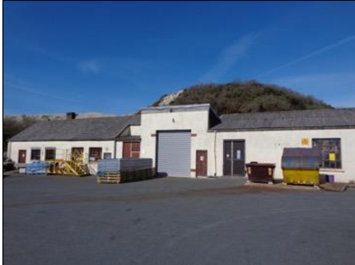
Figure 1. Building viewed from the south-east
