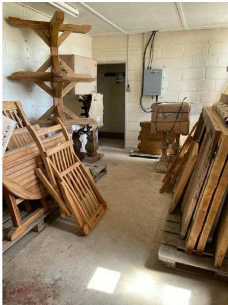
PHOTOGRAPH 8: Interior showing storage use and solid concrete flooring
