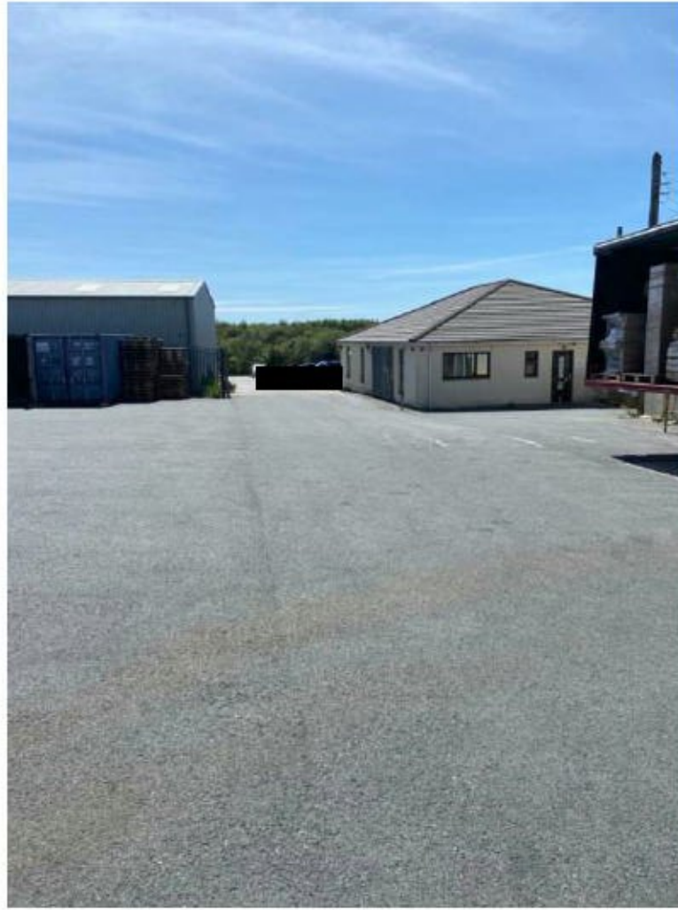
PHOTOGRAPH 1: Site access and tarmac parking and turning area
