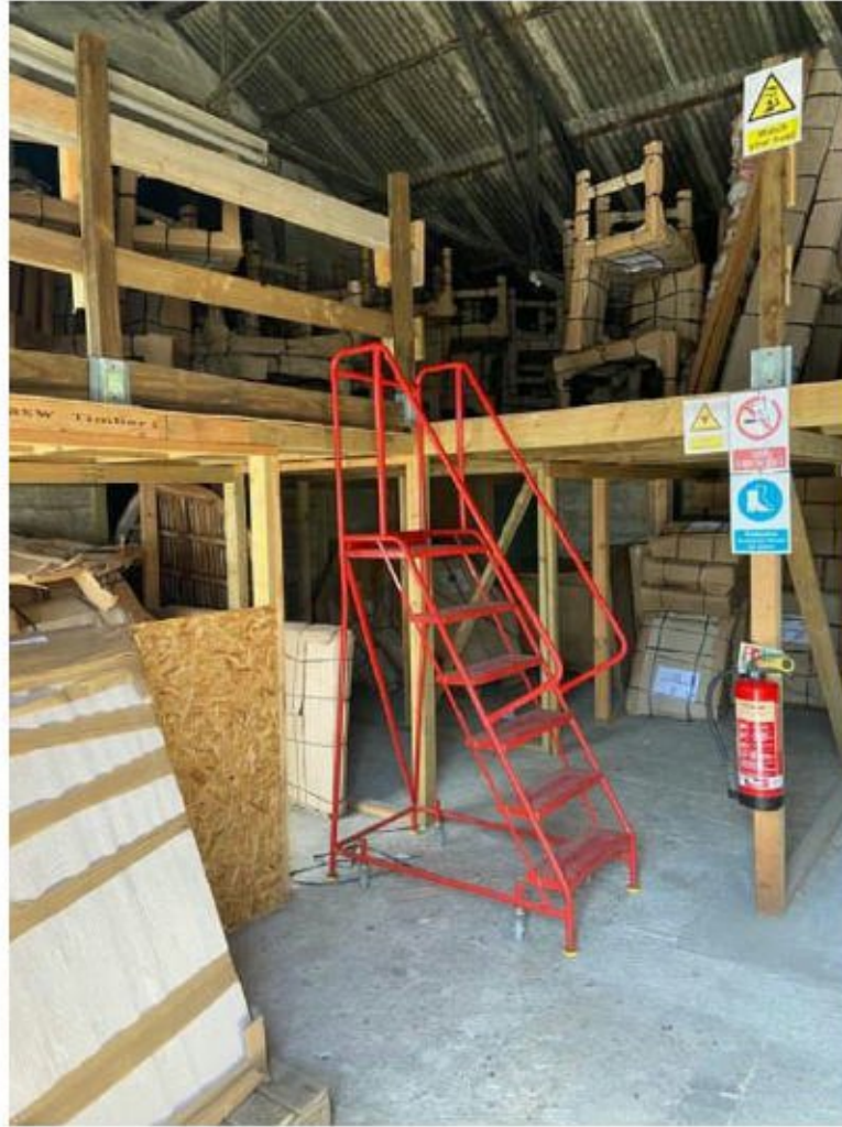
PHOTOGRAPH 7: Interior showing storage use and solid concrete flooring
