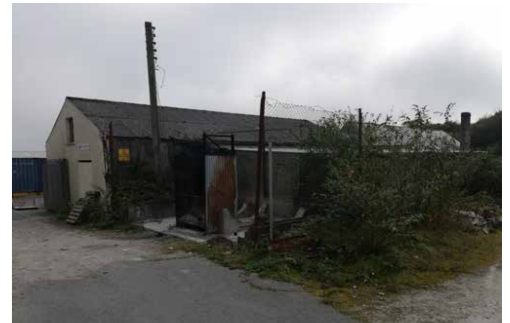
Rear side / gable elevation and overgrown nature of existing boundary treatment
