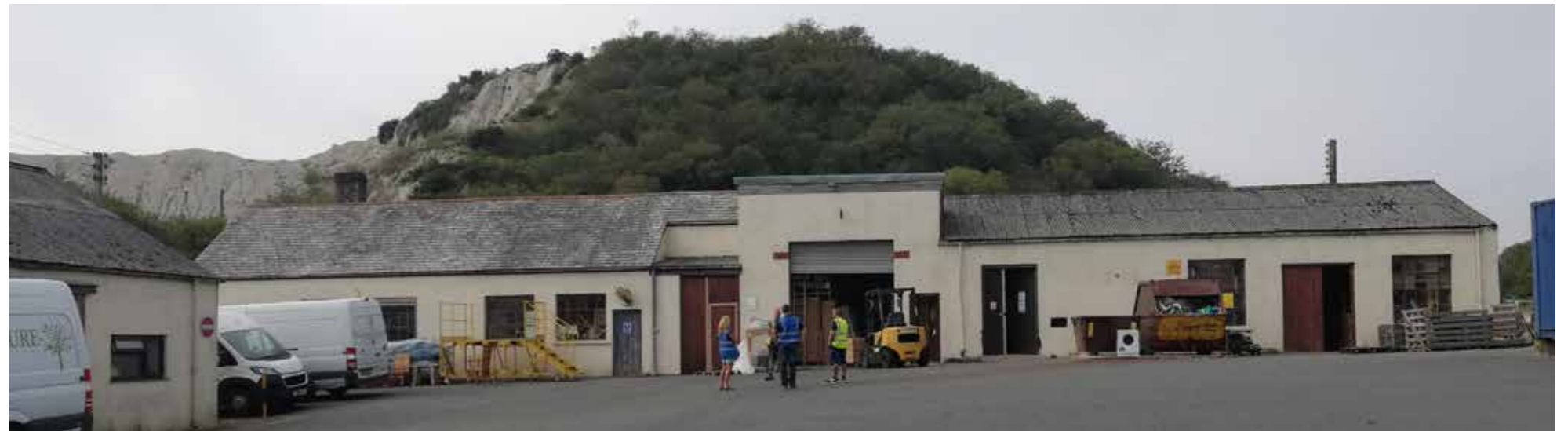
Existing front elevation with spoil heap behind being re-planted
