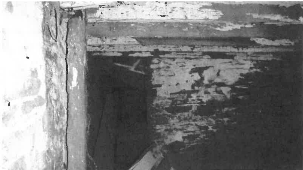
Photograph 4 Internal stone wall at ground floor level
