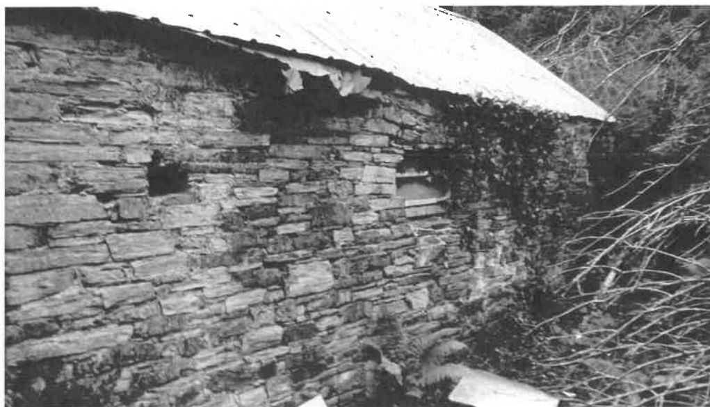
Photograph 5 Stonework to the east elevation flank wall above first floor level
