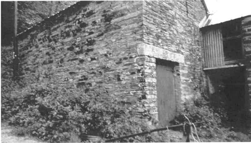
Photograph 1 South and west elevations
