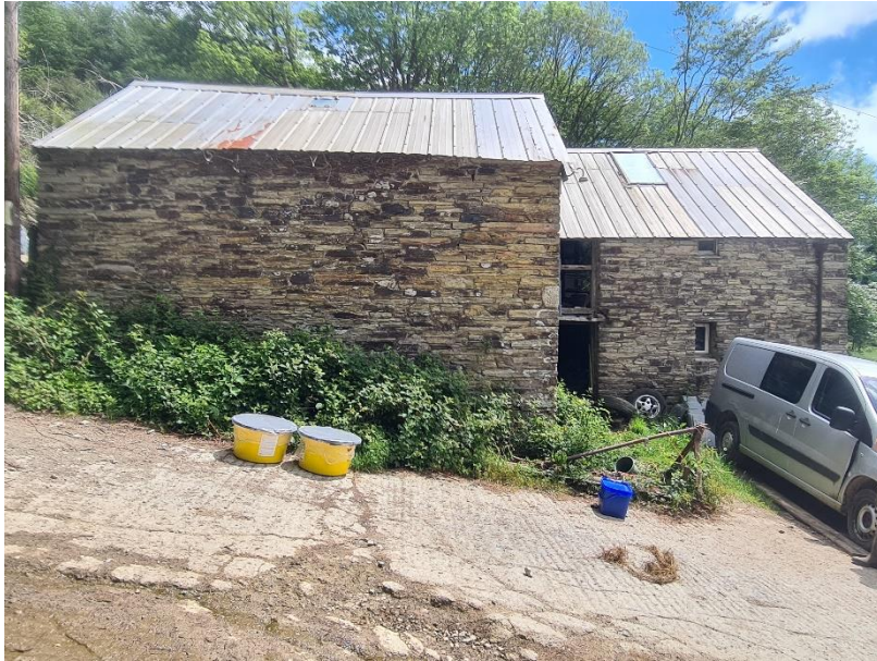
Looking South-east at front of barn
