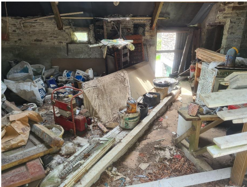
First floor interior
