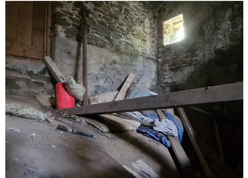
First floor interior
