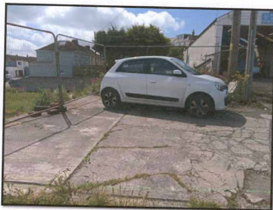
Photograph 10 – View from northwestern corner, looking south.
