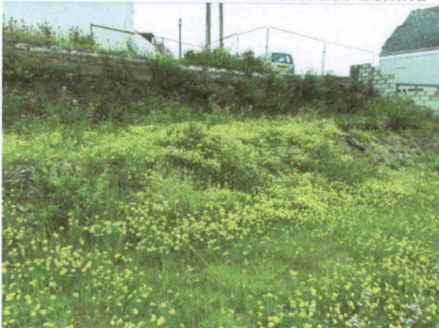
Plate 3. Embankment with rockface behind
