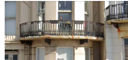
EXISTING CURVED STEEL RAILING
