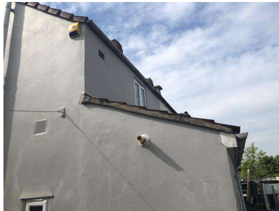
Side/Rear Elevation Viewed from Yard
