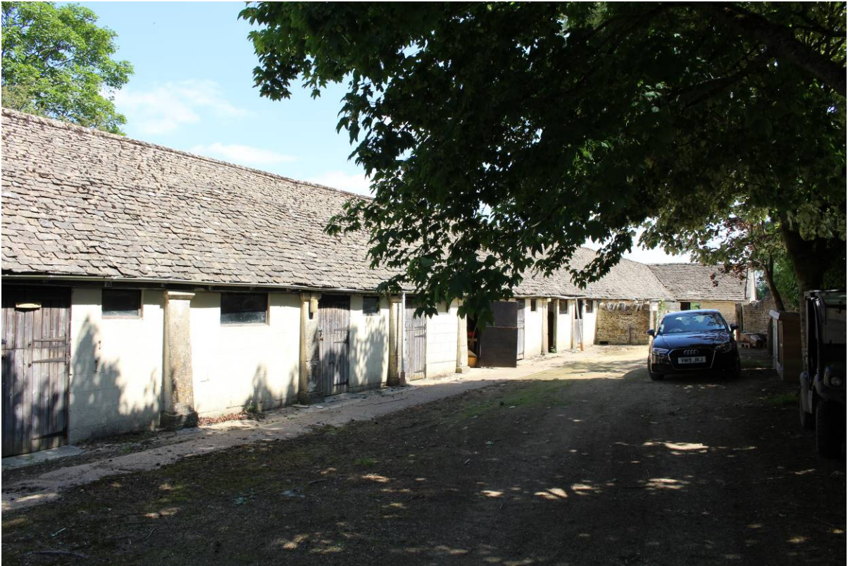
Image EDP 1: View of the former shelter shed, looking south-east showing the later infilling as stables.
