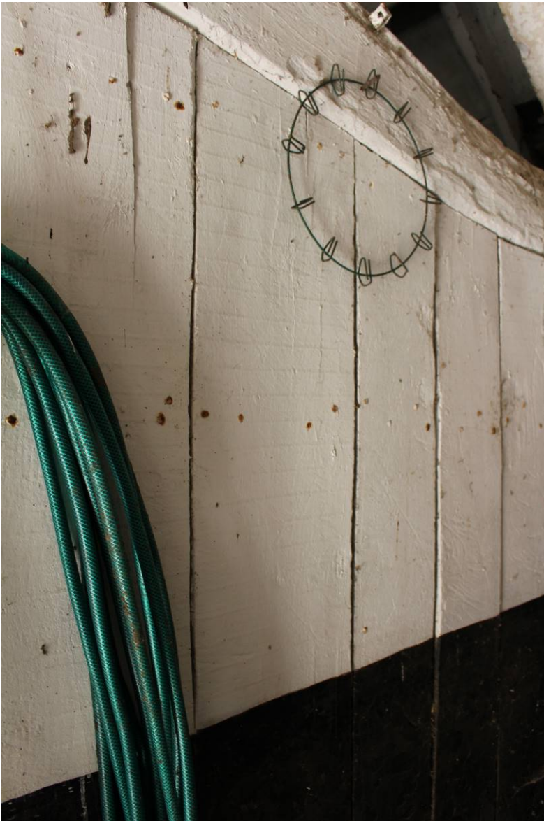
Image EDP 9: Close up of the internal partition boards, showing the clear machine marks.
