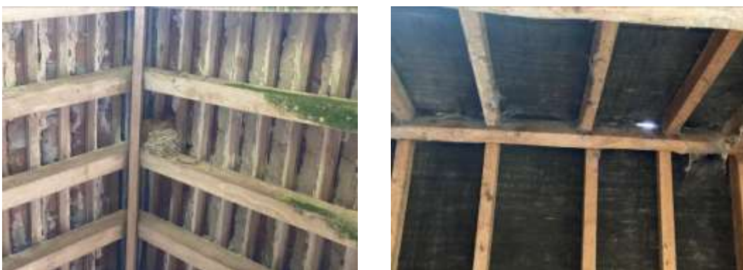
Figs. 20 & 21 Underside of roof
