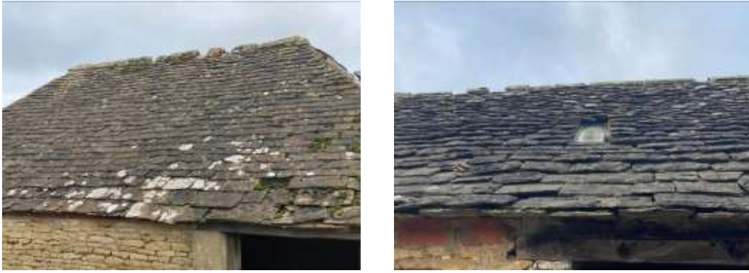
Figs. 17 & 18 Ridge and roof tiles
