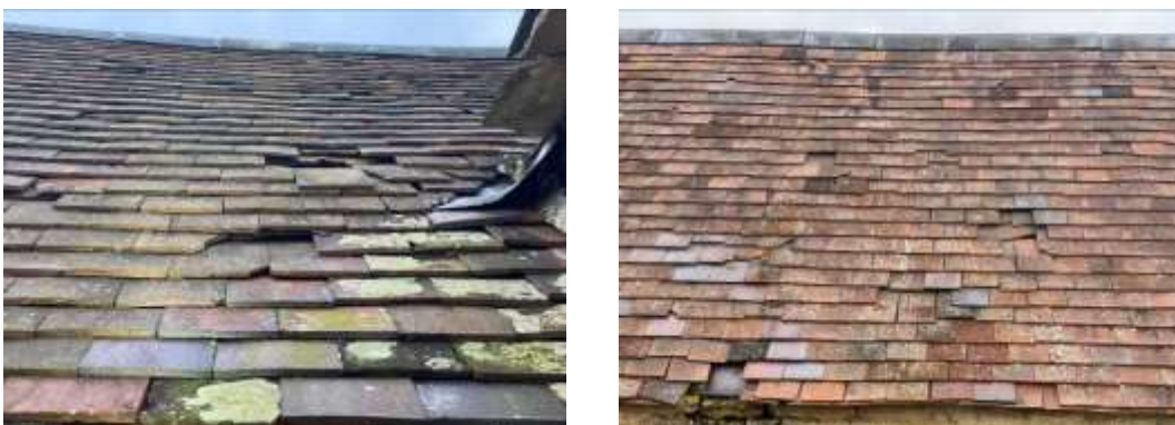
Figs. 15 & 16 Ridge and roof tiles
