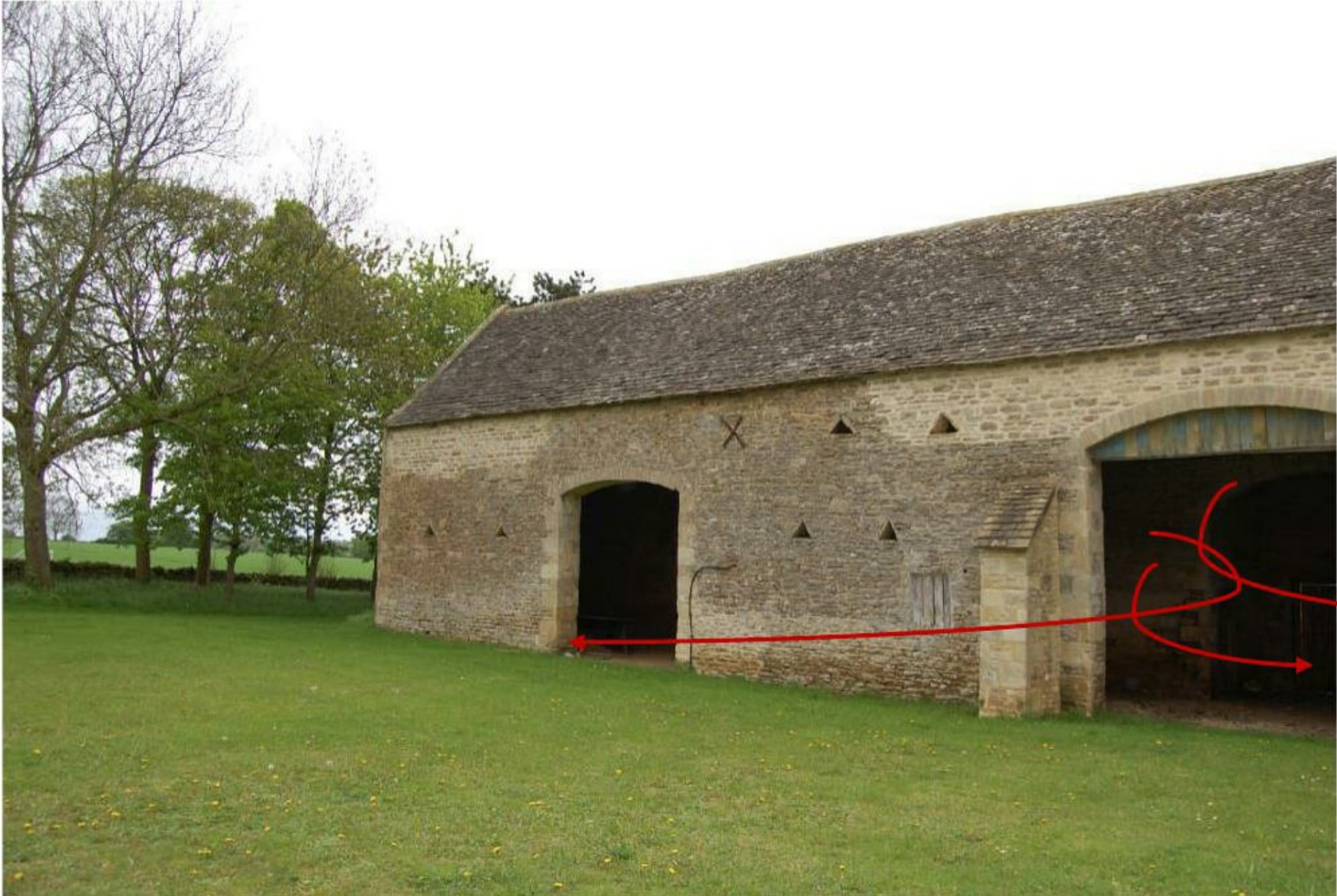
Figure 20. Photograph showing the emergence points of three common pipistrelle bats (red arrows). 12 th September 2019
