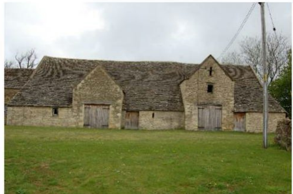
Photograph 4. Barn 1 viewed from the south-west.
