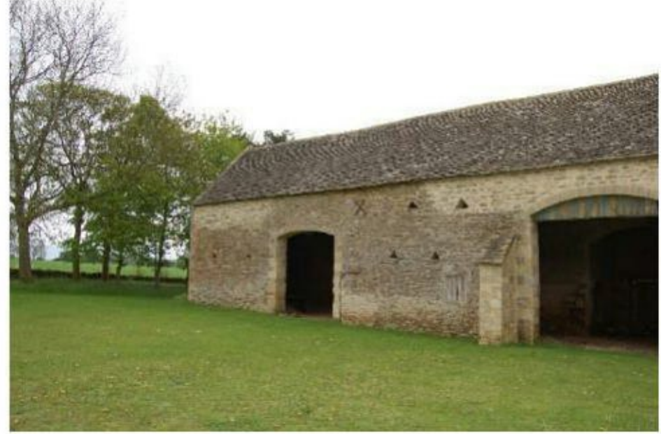
Photograph 2. The south-east end of the north-east elevation of Barn 1.
