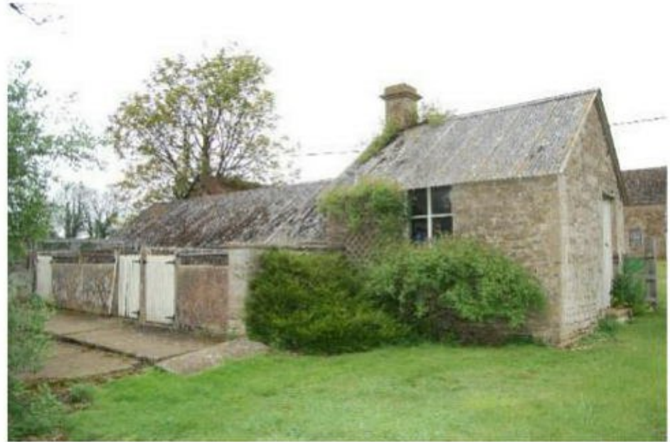
Photograph 16. The south-west elevations of the chicken sheds and potting shed-Barn 2.
