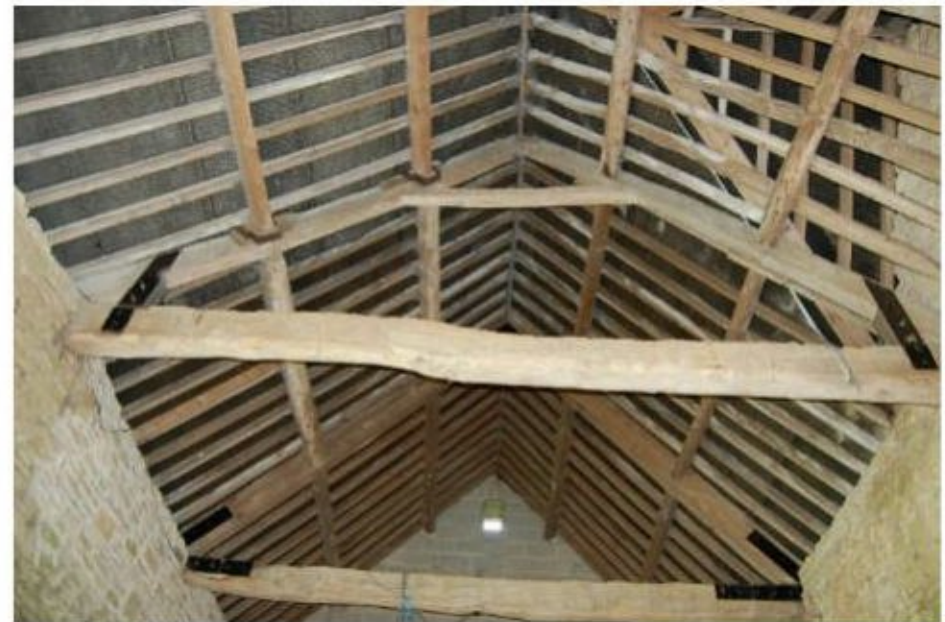
Photograph 6. The interior of the main barn (Barn 1).
