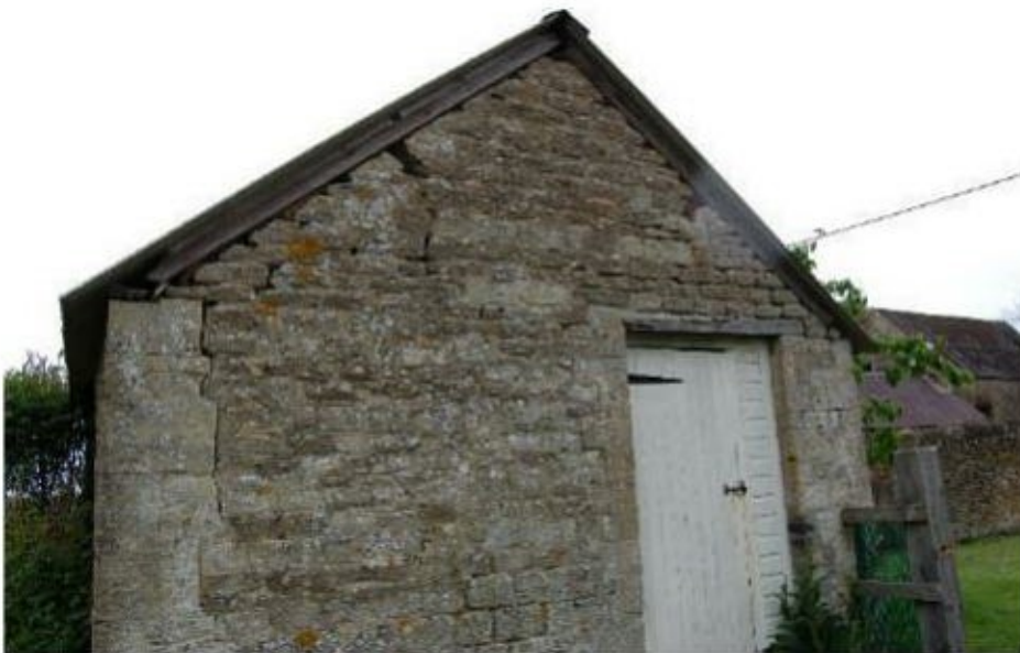
Photograph 17. The south-east elevation of the potting shed-Barn 2.
