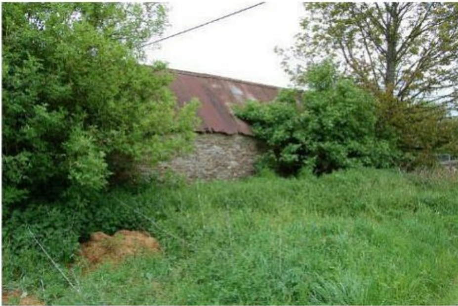
Photograph 15. The rear (north-west) elevation of the livestock shed-Barn 2.
