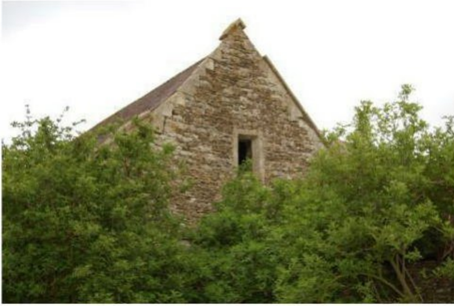
Photograph 13. Photograph of the south-west gable end of Barn 2-main barn.
