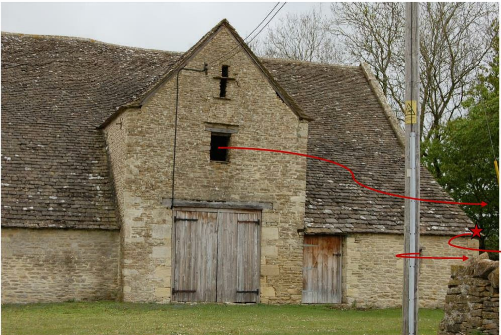
Figure 16. Photograph showing the roost locations (red stars) and emergence points (red arrows) of three of the common pipistrelle bats. 31 st July 2019.
