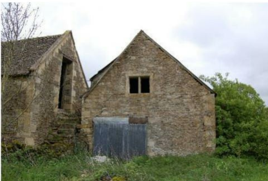
Photograph 11. The north-east elevation of Barn 2-main barn.
