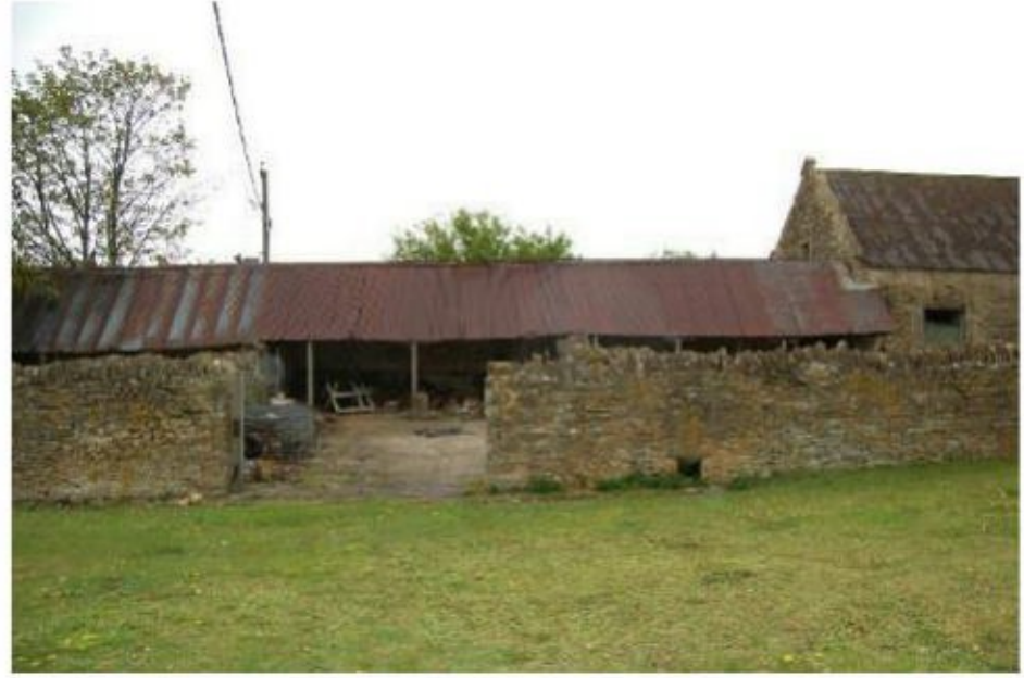
Photograph 14. Photograph showing the south-east elevation of the livestock shed- Barn 2.
