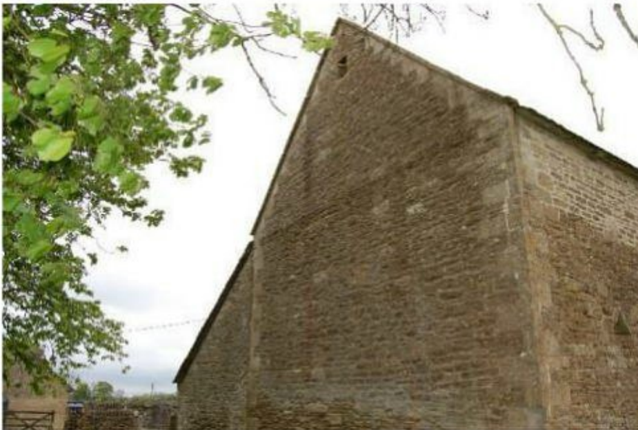
Photograph 3. The south-eastern gable of Barn 1.
