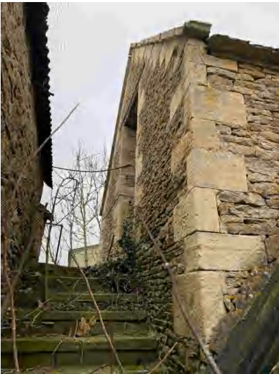
3.24 West elevation of Building B (DIA).
