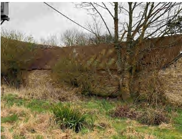
3.56 The rear (west elevation) of Building D (DIA).
