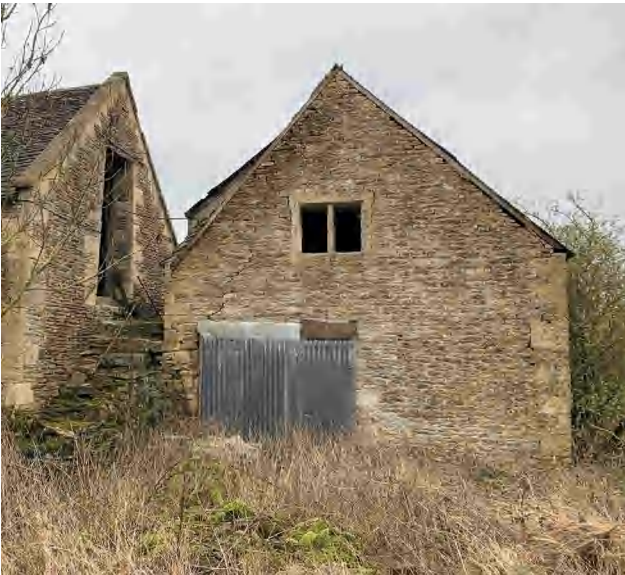
3.41 The north elevation of Building C (DIA).
