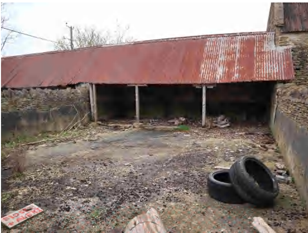
3.54 Building D, north end (DIA).
