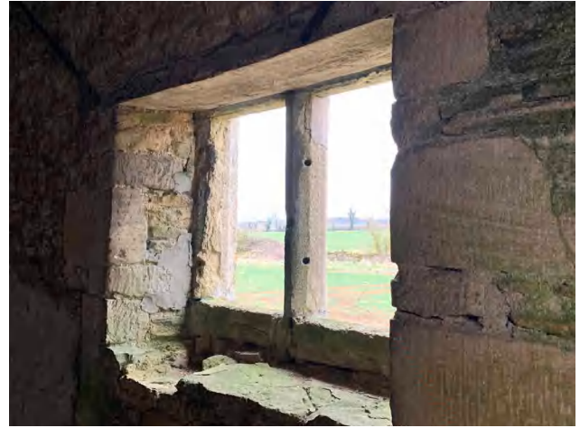
3.47 Window in northern gable of Building C, from within (DIA).
