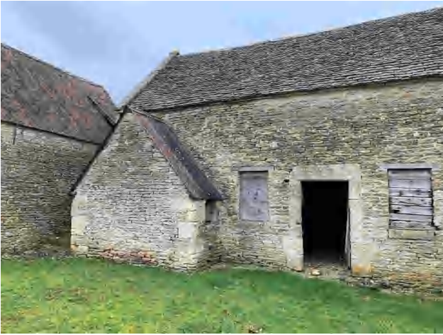
3.27 Building B, south elevation (DIA).
