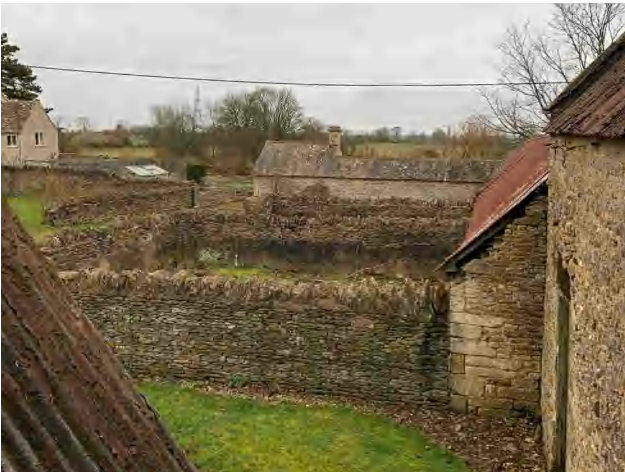
3.62 The enclosures in front of Building C, from the north (DIA).
