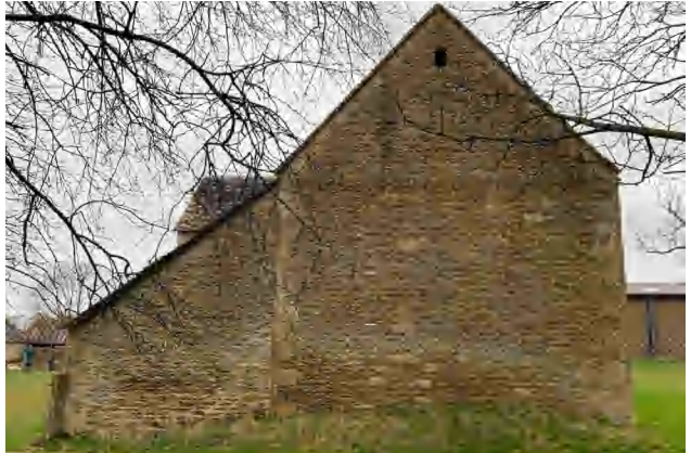
3.3 Building B, east elevation (DIA).
