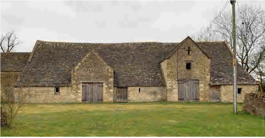
3.5 Building A, south elevation (DIA).
