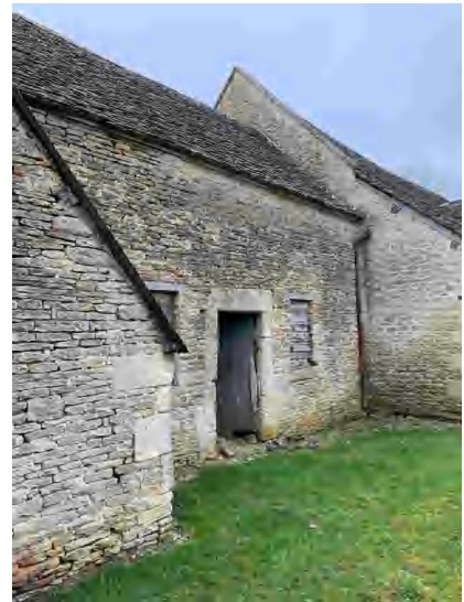
3.26 Building B, south elevation, from the south west (DIA).
