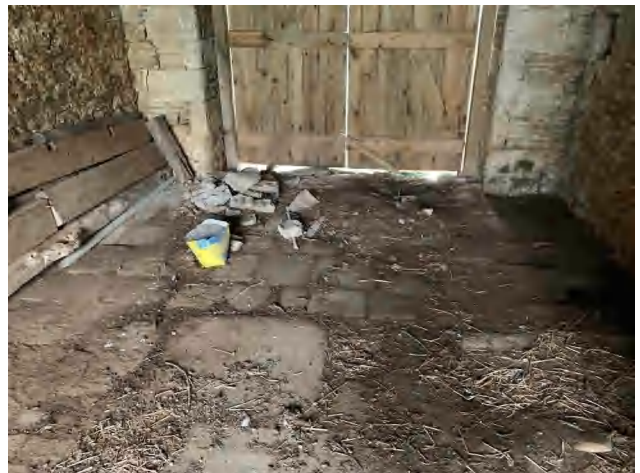
3.19 Stone flagged floor in the southern porch of the eastern part of Building A (DIA).
