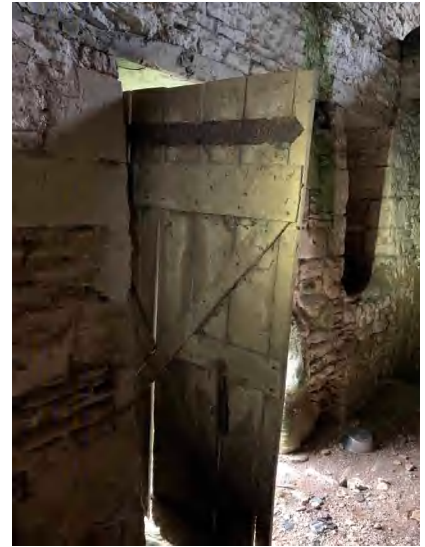
3.32 Inside of door to building B (DIA).
