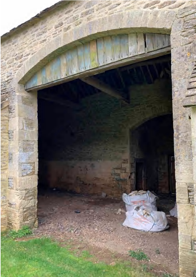
3.2 Building A, north elevation, detail of west door (DIA).
