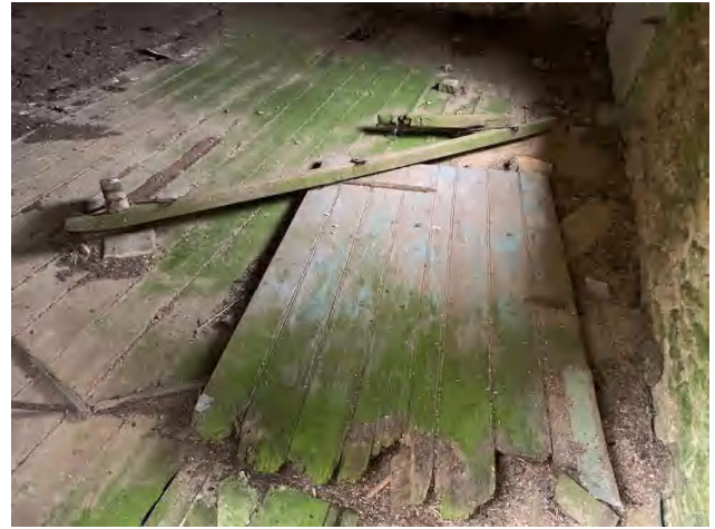
3.49 Former door to the first floor of Building C (DIA).
