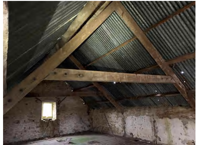
3.52 Roof of Building C, looking east (DIA).
