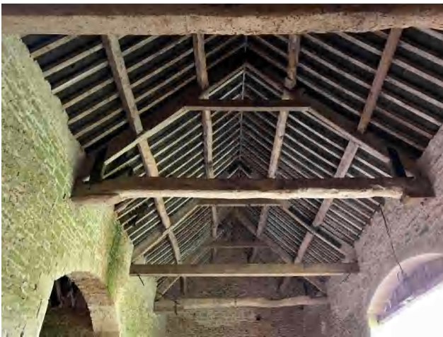
3.10 Building A - the roof of the western part, looking west (DIA).
