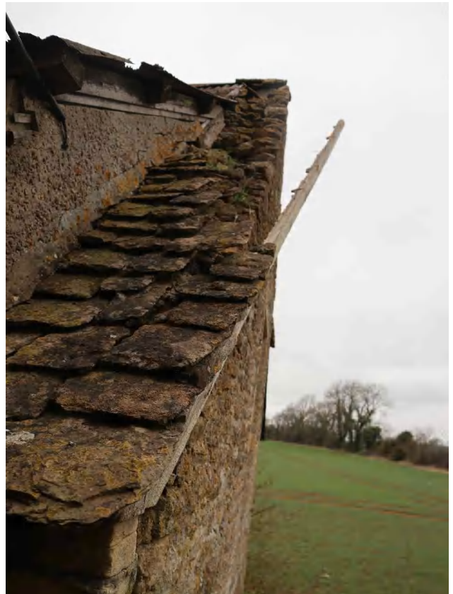
3.50 Remaining area of stone slate on northern gable wall of Building C (DIA).
