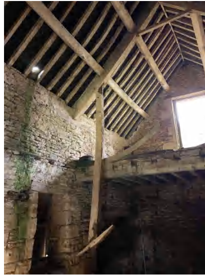
3.30 Building B, interior looking south west (DIA).
