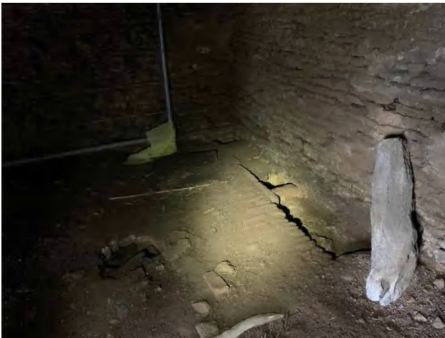
3.34 The floor in the north western corner of Building B (DIA).
