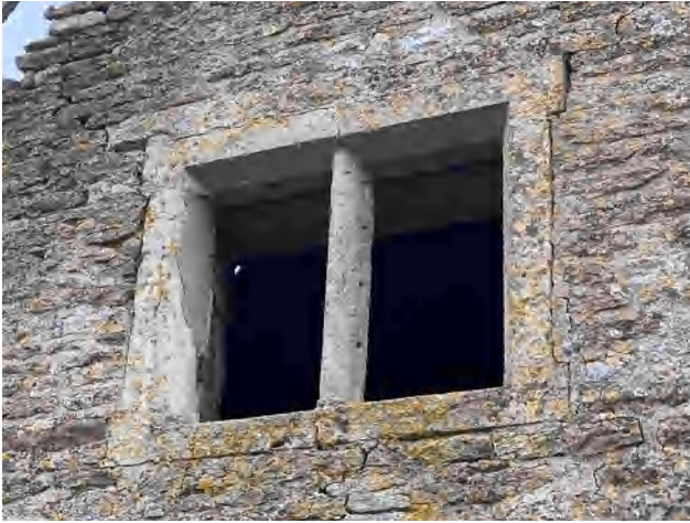
3.46 Stone mullion window in northern gable of Building C (DIA).
