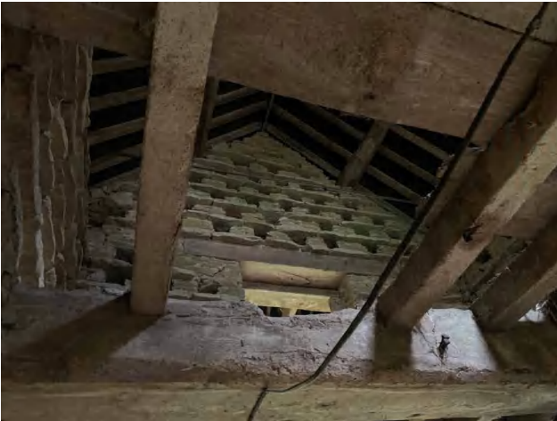
3.21 Building A, east end. View up from ground level into the pigeon house, showing nest boxes built into the gable wall (DIA).
