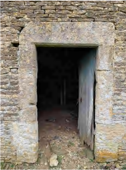
3.28 Building B, door in south elevation (DIA).
