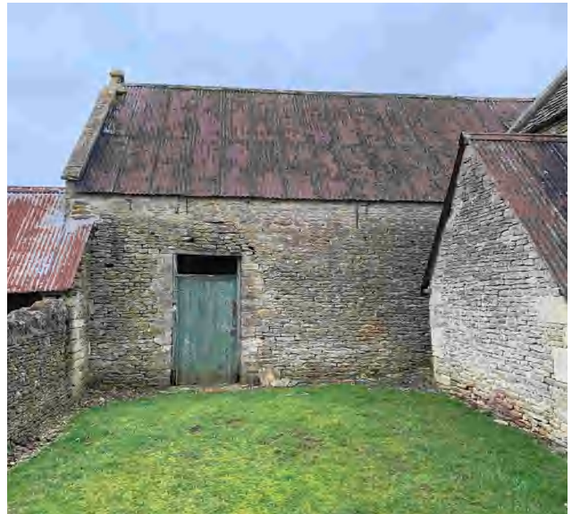
3.44 East elevation of Building C (DIA).
