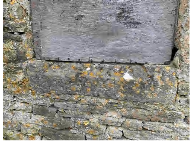
3.29 Building B, south elevation - detail of window cill (DIA).
