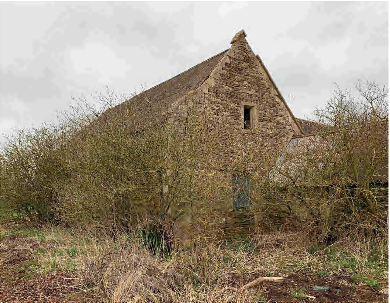
3.40 The south elevation of Building C, from the south west (DIA).
