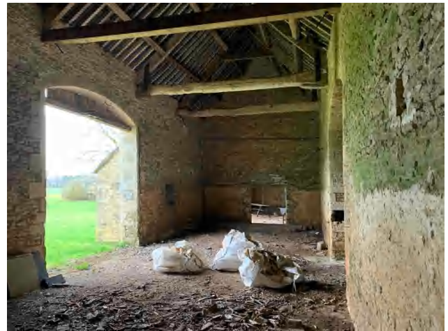
3.9 Building A - the western part, from the south west (DIA).
