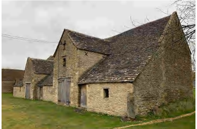
3.4 Building A, south elevation, from the south east (DIA).
