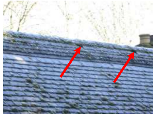
Figs. 5 & 6 Roof of chapel and missing tiles (arrowed)
