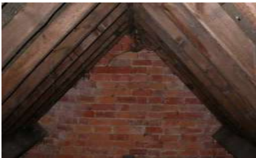
Figs. 27 & 28 Roof void with horizontal gap in felt (arrowed)
