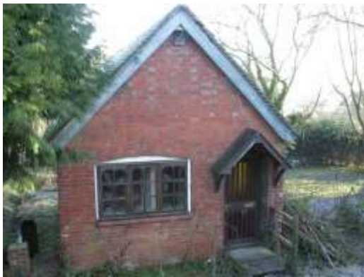
Figs. 7 & 8 West gable end showing barge boards and cavity in roof end
