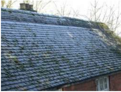
Figs. 5 & 6 Roof of chapel and missing tiles (arrowed)
