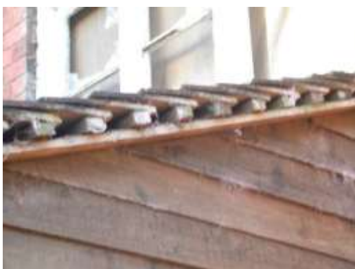
Fig. 13 Porch roof end
