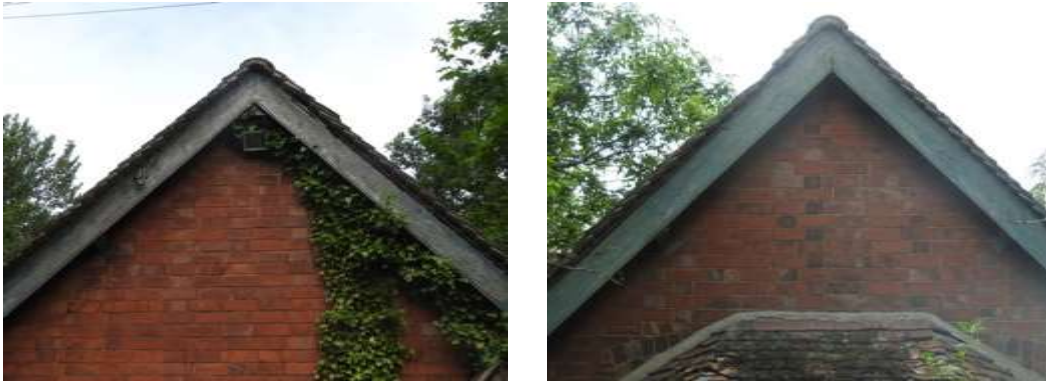
Figs. 33 & 34 Gable ends – with west gable gaps (L) and sealed east gable (R)
