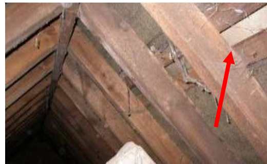
Figs. 27 & 28 Roof void with horizontal gap in felt (arrowed)
