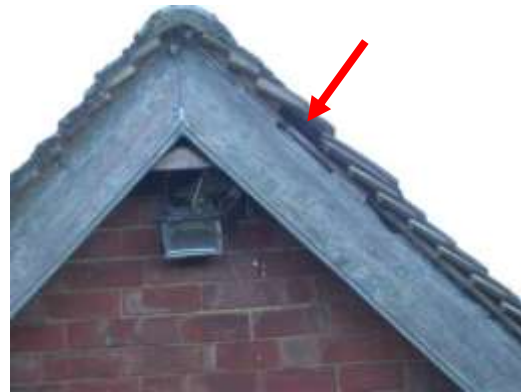
Figs. 7 & 8 West gable end showing barge boards and cavity in roof end
