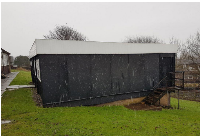
Existing Outbuildings to the West
