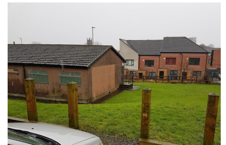
Existing Outbuildings to the West
