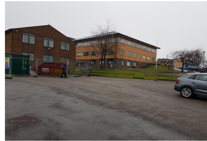
Existing school buildings and parking
