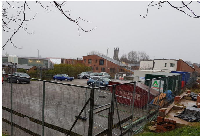
Existing temp fencing and units, to parking area
