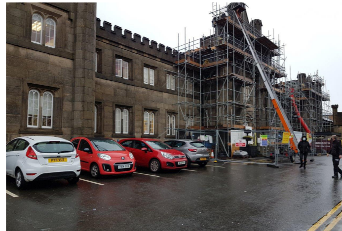
Existing School with adjacent parking
