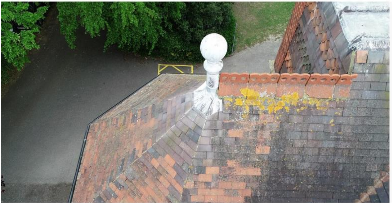
Ridge Tiles- Existing
