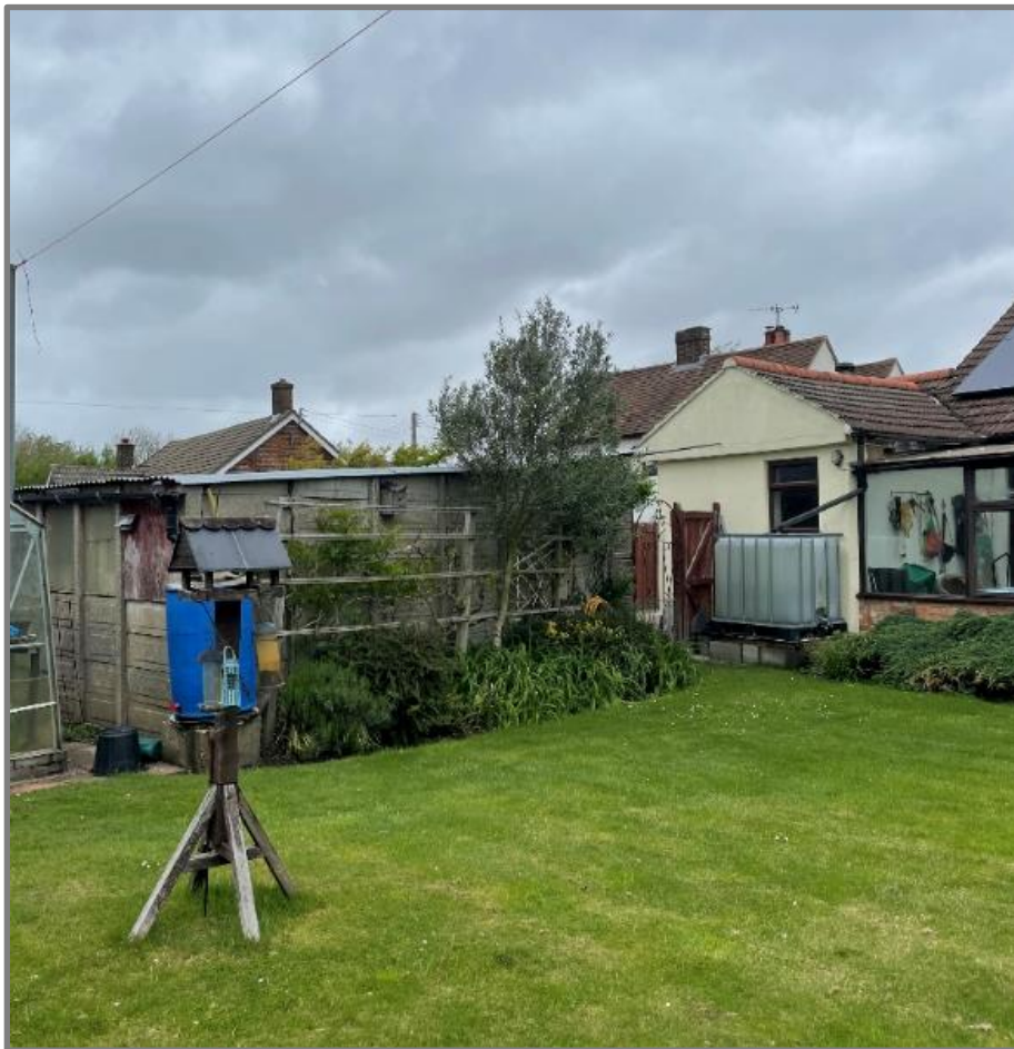
10. Existing outbuilding structures in rear garden
