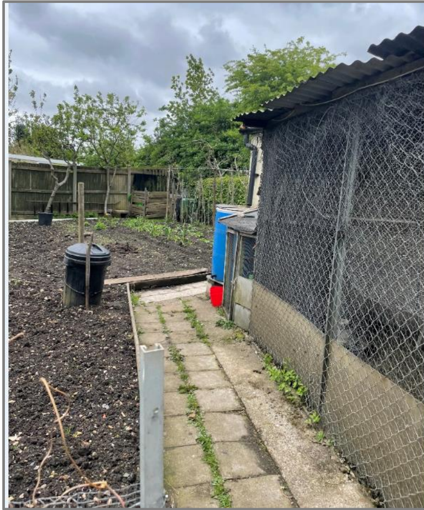
11. Existing outbuilding and shed structures in rear garden
