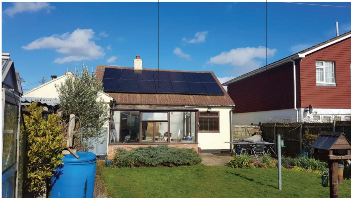
4. Existing bungalow as viewed from the rear garden
