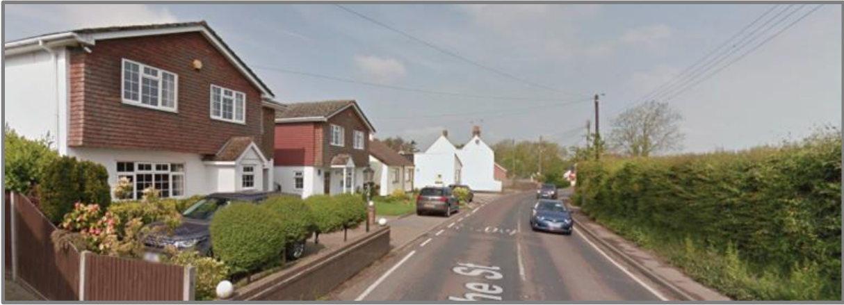
9. Existing bungalow as viewed from The Street, showing neighbouring two storey properties 'Stonechats' in foreground
