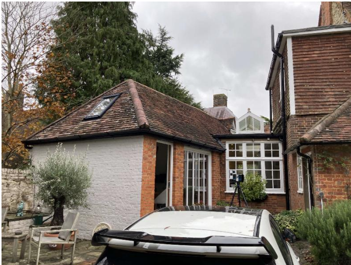
Fig 6. Rear of kitchen and dining room wing
