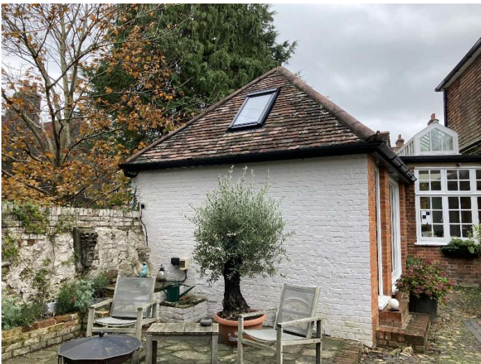
Fig 7. Condition of existing dining room exterior
