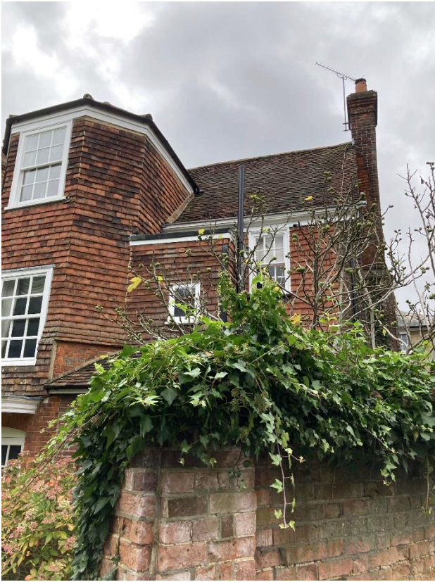
Fig 8. Rear flat roof extension at first floor
