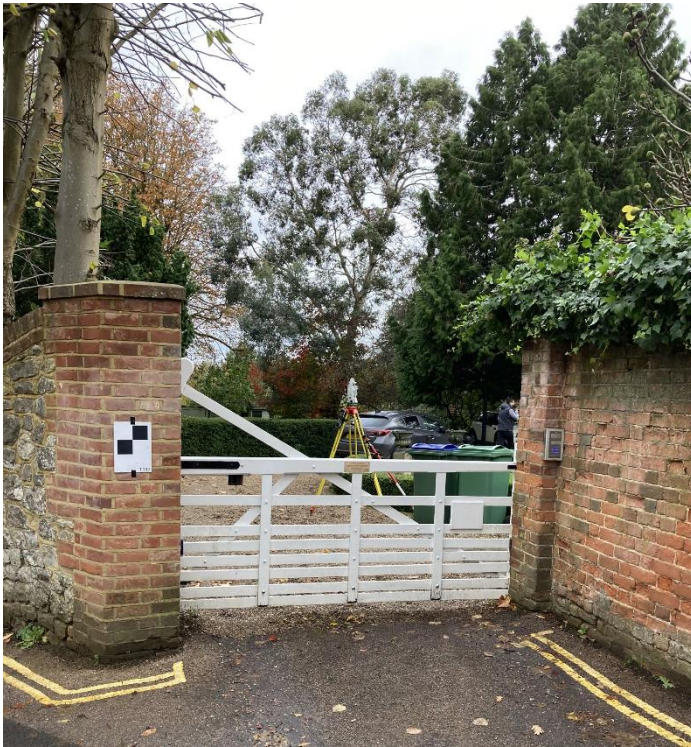
Fig 9. Existing rear car access gate
