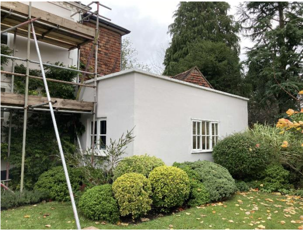
Fig 3. Existing front facing single storey extension
