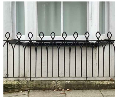
Existing railings at no. 12 High Street opposite
