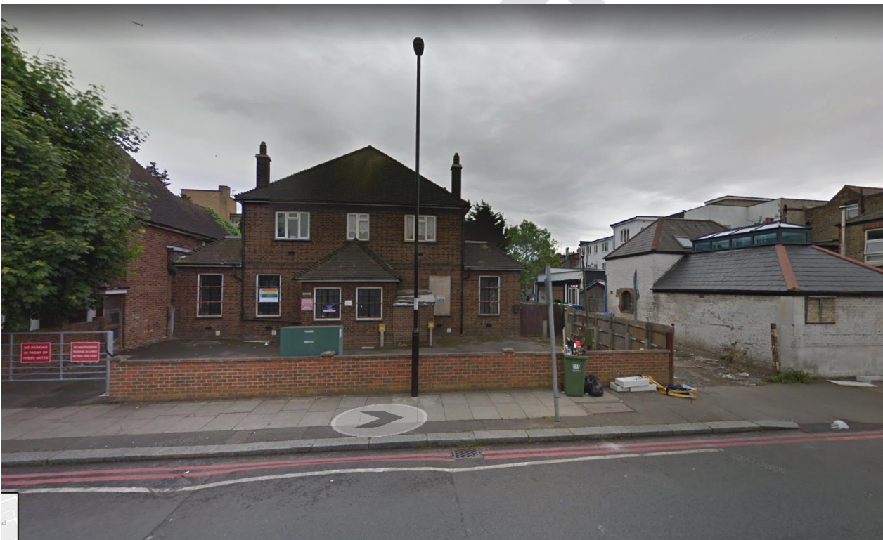
Photo 2 -4 Bellingham Road-prior to development
