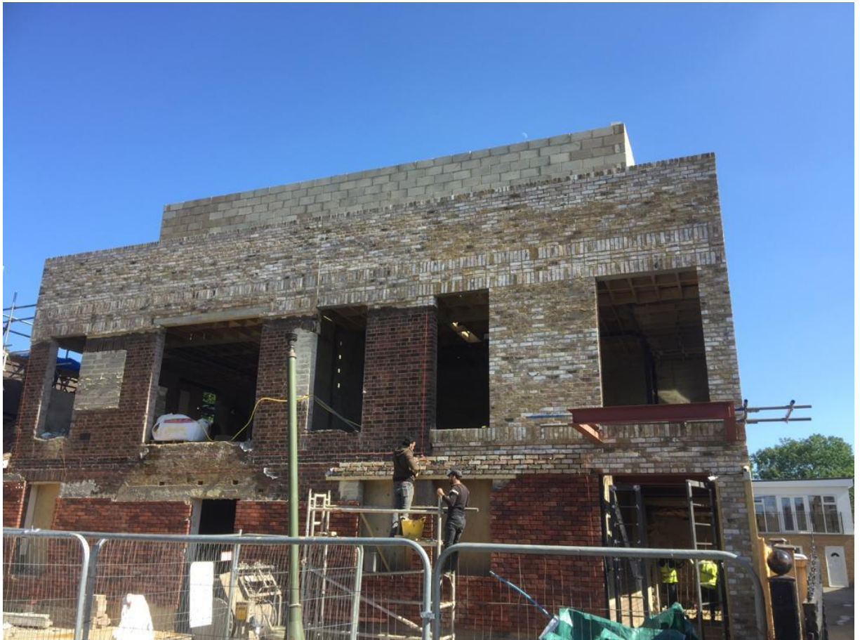
Photo 3 Number 4 Bellingham Road under construction
