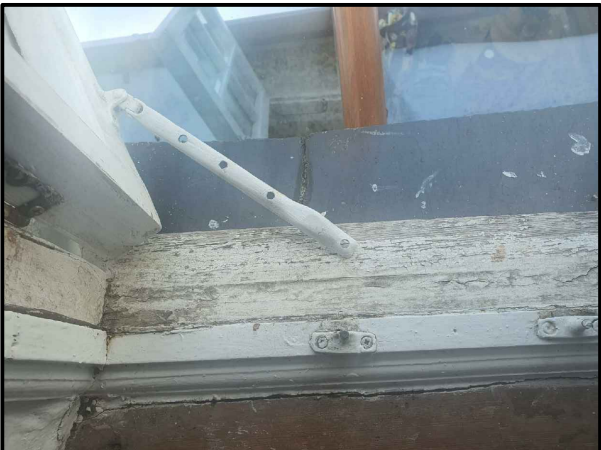
(Sc) PHOTOGRAPHY SHOWING TYPICAL WINDOW DILAPIDATION - TAKEN JULY 2021 NTS @ A3
