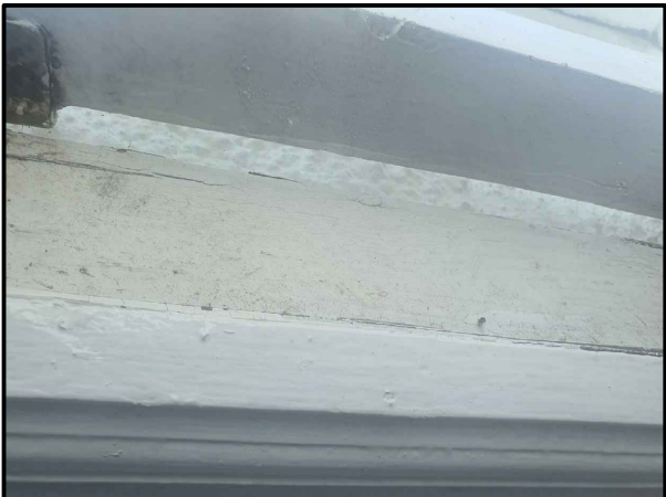
(Sc) PHOTOGRAPHY SHOWING TYPICAL WINDOW DILAPIDATION - TAKEN JULY 2021 NTS @ A3
