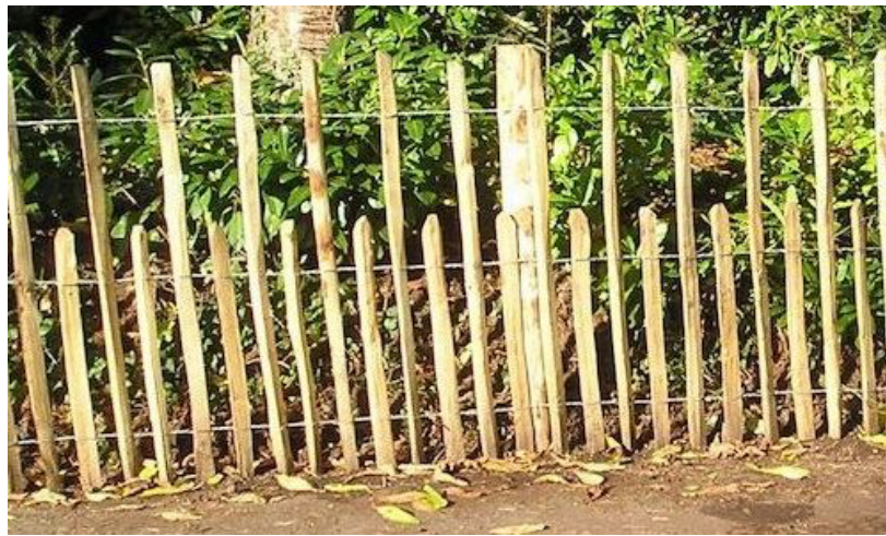
Chestnut pale fencing erected around every tree at least to extent of canopy spread, min 1.2m high
