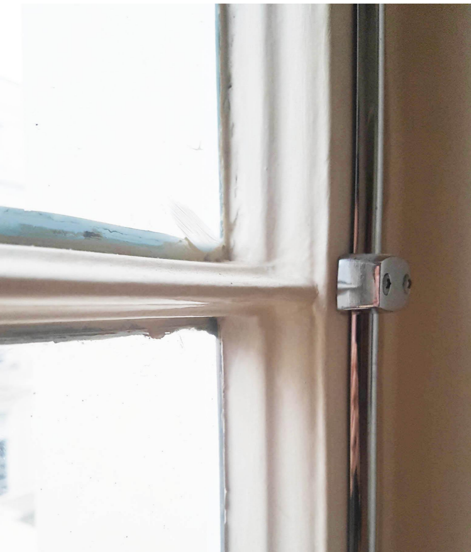
EXISTING GLAZING BAR AND WINDOW FRAME
