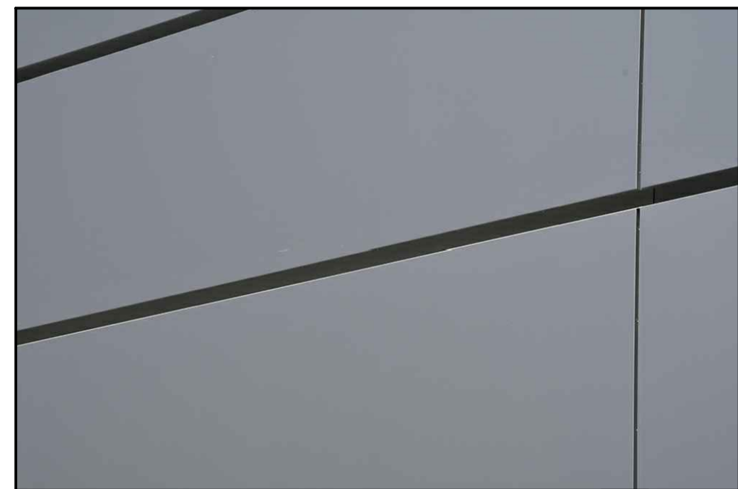
Alucabond Showroom facade cladding Finished in RAL 9006 Silver
